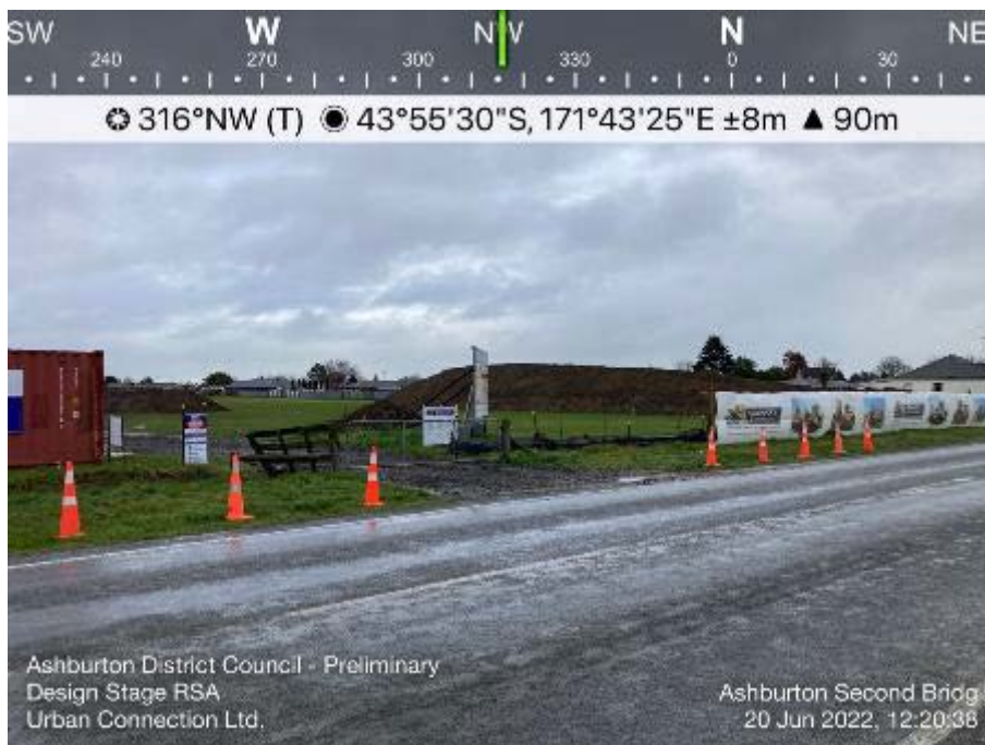
Figure 2-24 - New Subdivision on Grahams Road Under Construction
