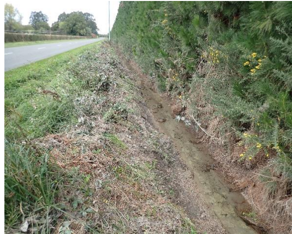
Figure d. Looking downstream at the dredged section of Willowby Water Race, flowing south along Longbeach Road.(photo 30 th April 2021).
