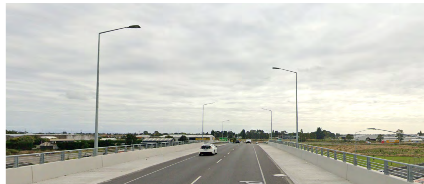
Figures 28 & 29: Alternating lighting fixed to piers on the Springs Road bridge, Christchurch Southern Motorway, Google Earth.
