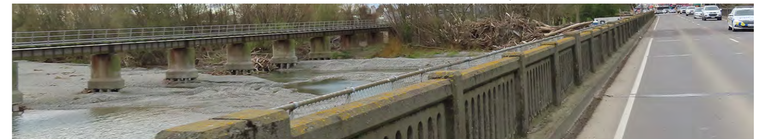
Existing SH1 Bridge parapet and rail bridge piers - https://www.ashburtondc.govt.nz
