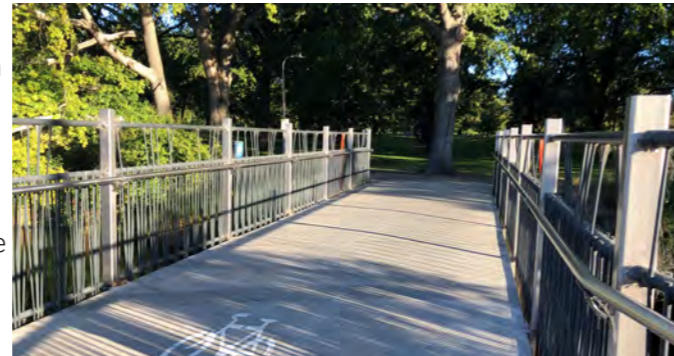
Hagley Park Bridge with cycle grab rail - author
