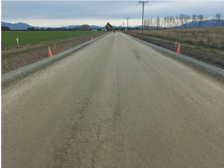
Lismore Mayfield Rd – prepared for sealing
