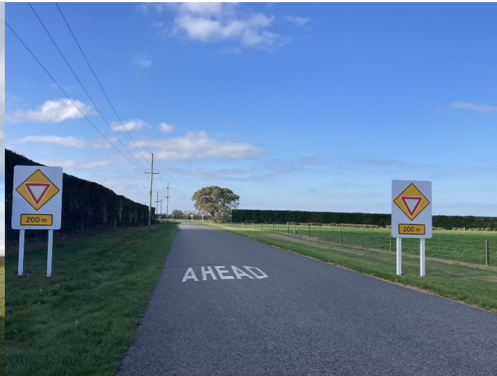
After – gated Give Way Ahead warning signs with white backboard
