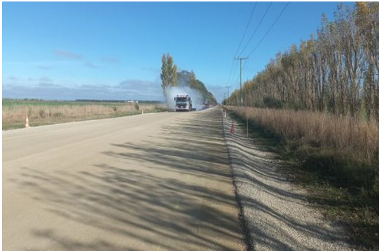
Thompsons Track – sealing in progress
