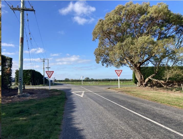
After – gated Give Way Ahead warning signs with white backboard
