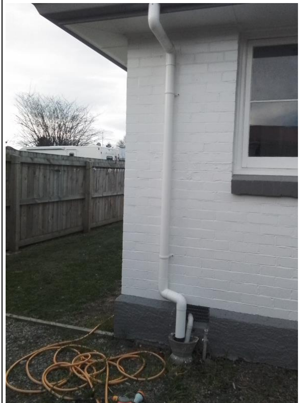
Example of Illegal Stormwater Connection (Tinwald)
