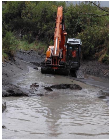
Pudding Hill intake silt removal
