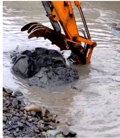
Pudding Hill intake silt removal
