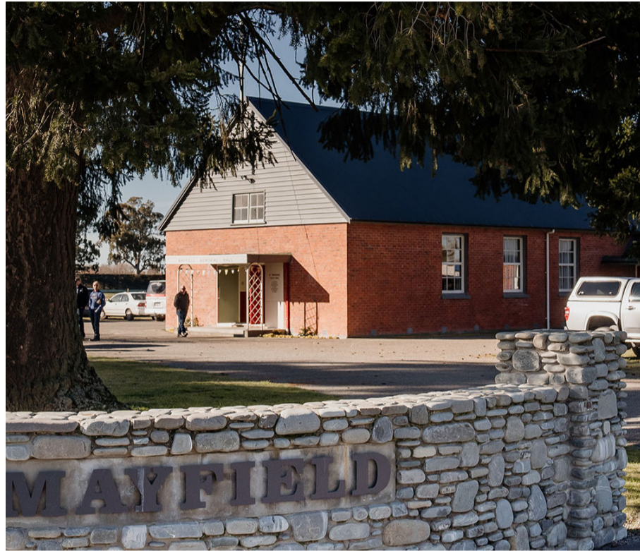
ABOVE: The Mayfield Memorial Hall was recently granted $10,000 to replace the entrance doors to the supper room.
