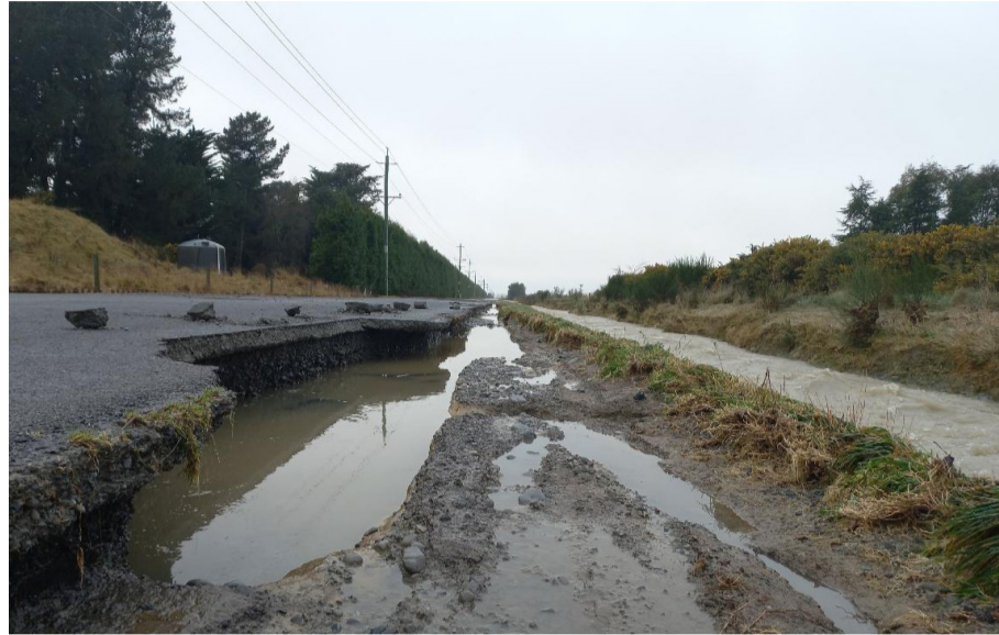
ABOVE: Methven Chertsey Road suffered major scours and damage. BELOW: The intersection of Thompsons Track and SH77.
