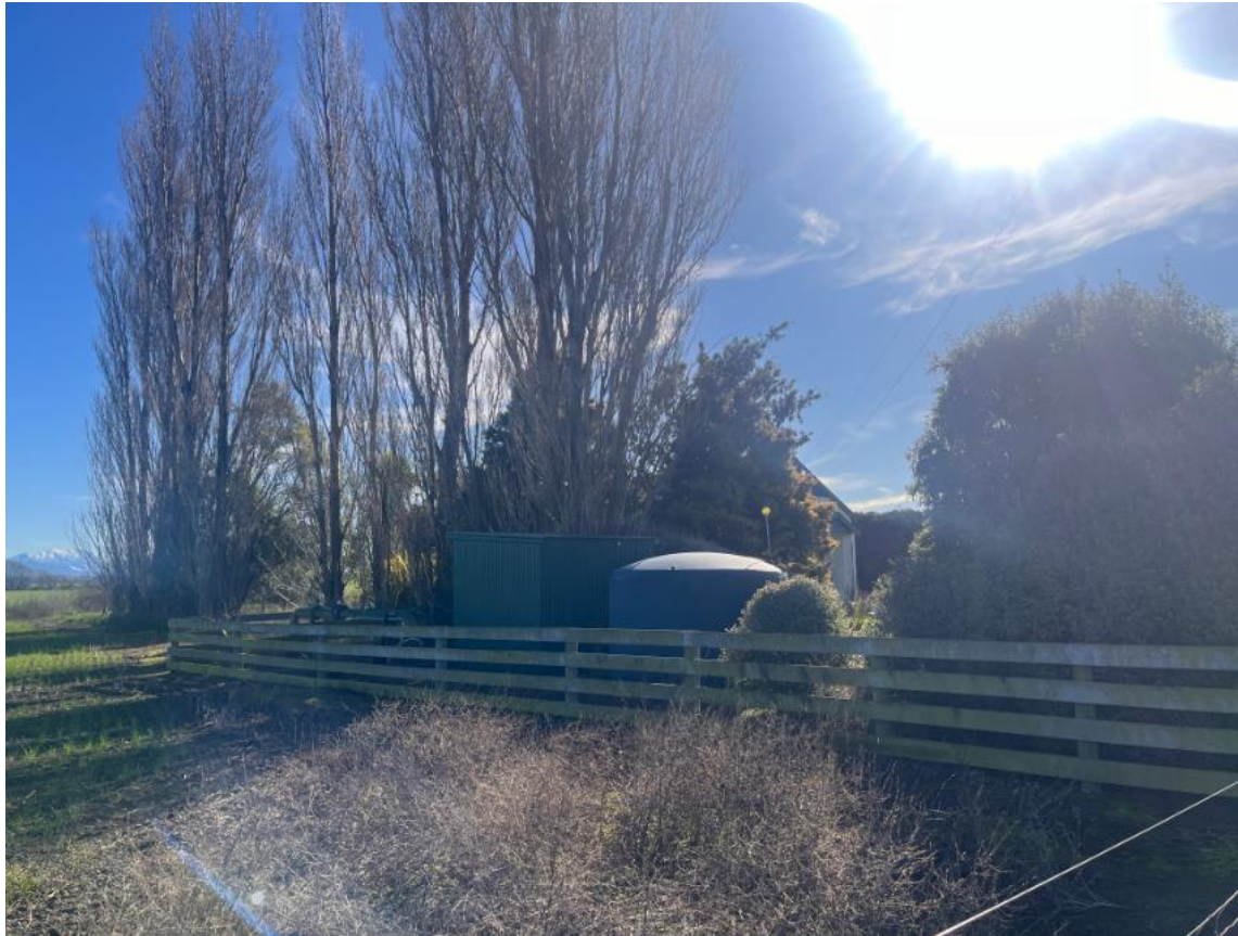
Figure 6. Pump station located at 902 Longbeach Road, southern boundary of Application Site
