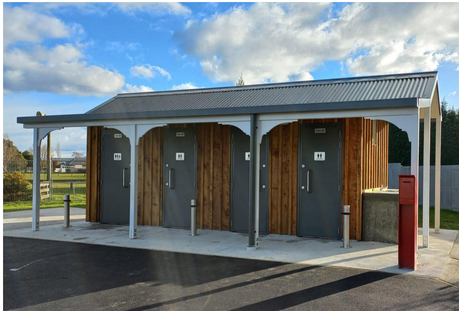
Construction of the new toilets at the Mayfield Domain has finished and the public conveniences are open for business.
