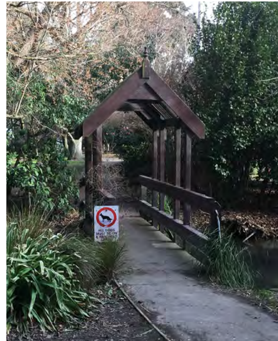
FOOTBRIDGE AT SPORTSFIELD END OF WATERWAY
