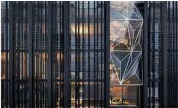
BLACK STEEL CLADDING AND FRAMING
