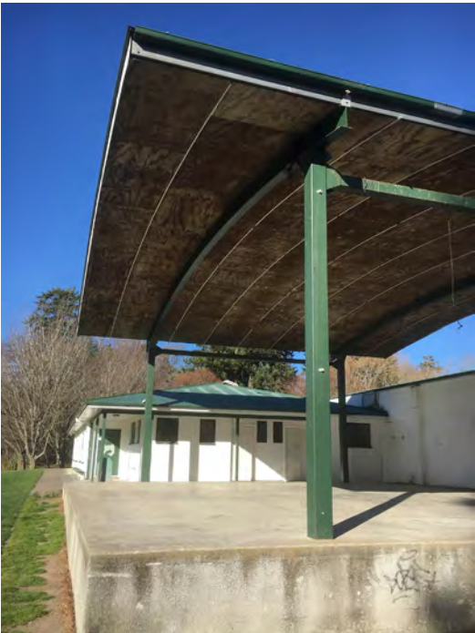
EXISTING COVER OVER PAVILION PERFORMANCE STAGE
