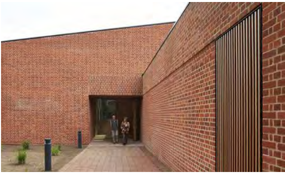
BRICK CLADDING, WALLS AND PAVING
