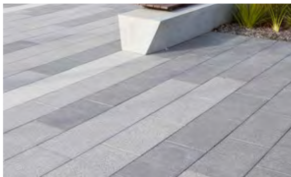
CONCRETE FEATURE PAVER'S
