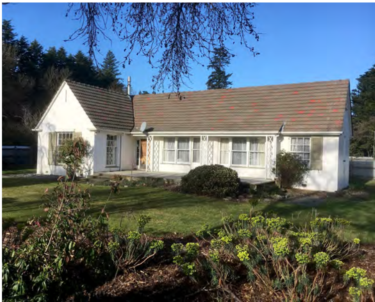
EXISTING CURATOR’S HOUSE
