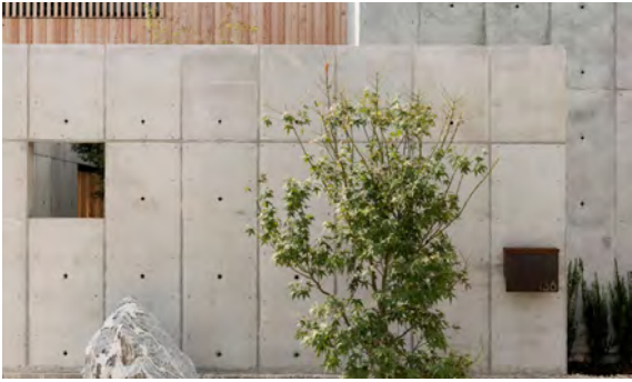
CONCRETE BUILDINGS, STRUCTURES AND PAVING
