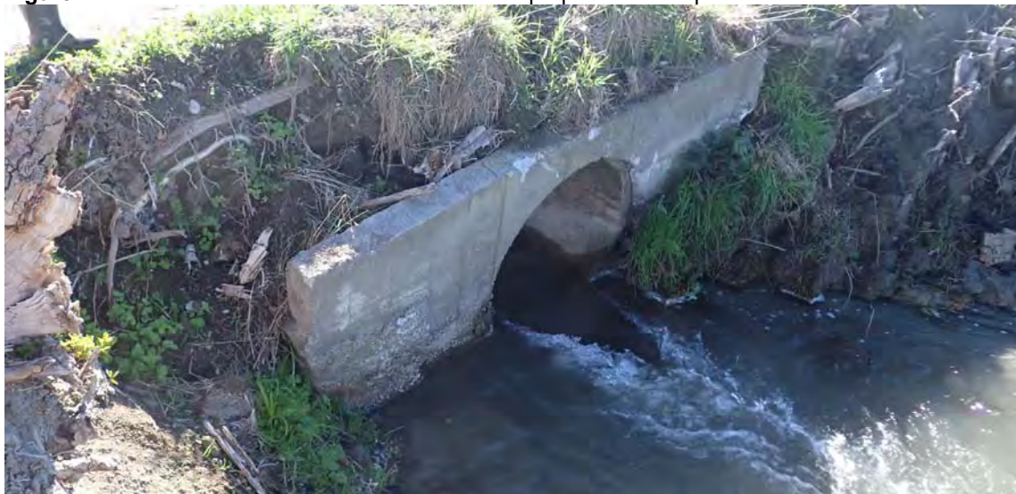
Figure iv. The existing culvert in the proposed development area. This culvert is too narrow and perched too high under the NES-F 2020
