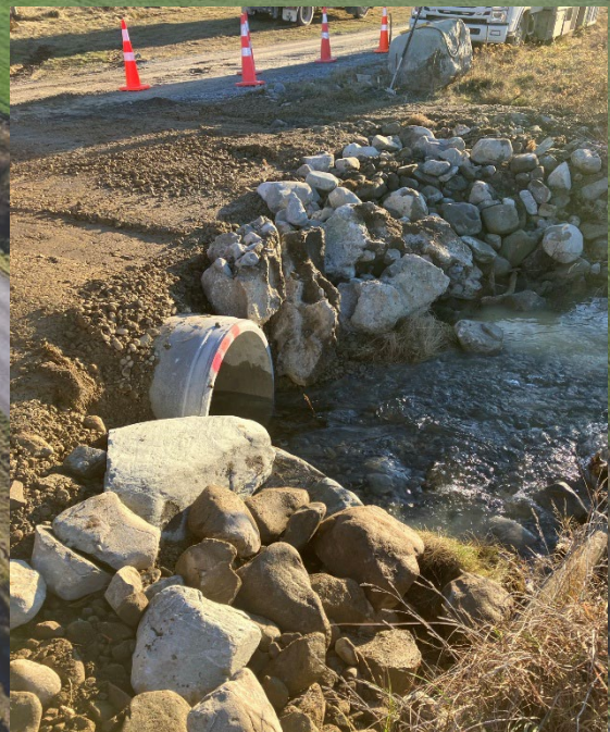
Culvert replacement on Hakatere Potts
