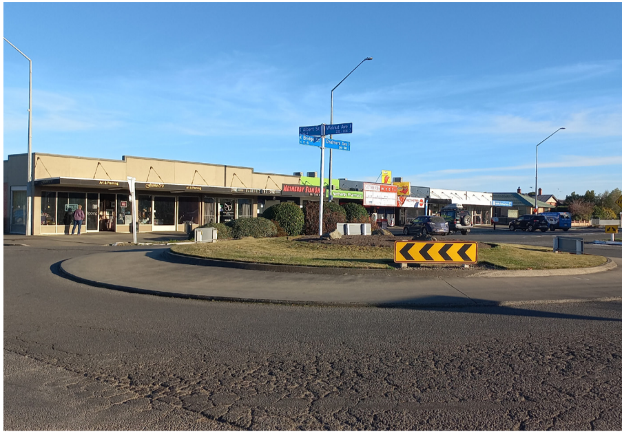
The Netherby roundabout at the intersection of Walnut Avenue and Chalmers Avenue will receive a new asphalt surface. Access to parks in front of shops remains.
