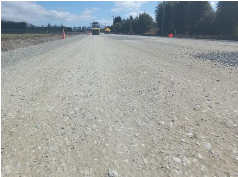
Ealing Montalto Road - prepared for sealing
