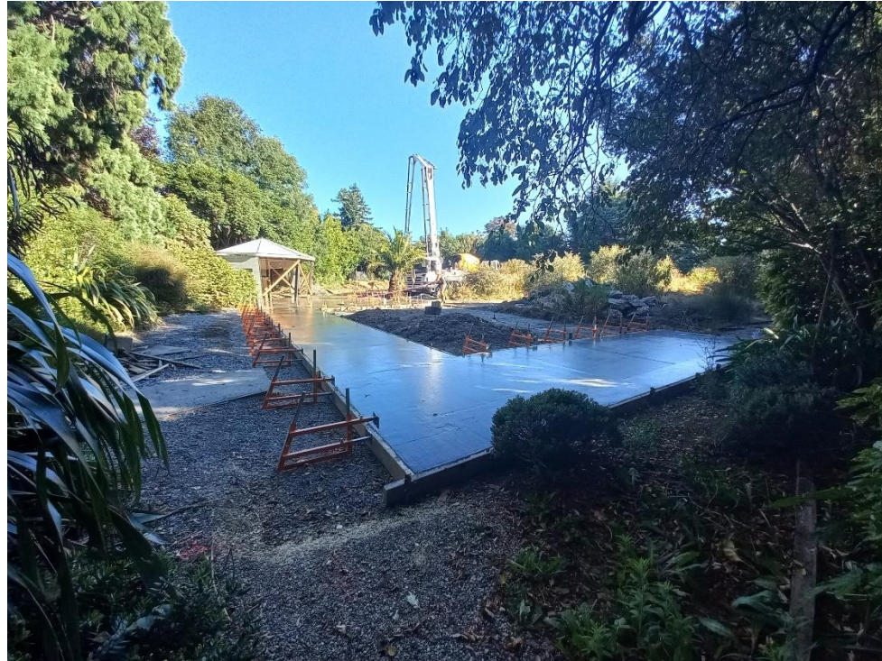
The new paths getting poured via a concrete pumping unit.
