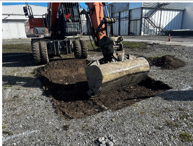
Photograph 9. View of TP16 showing demolition fill underlying the former trades building
