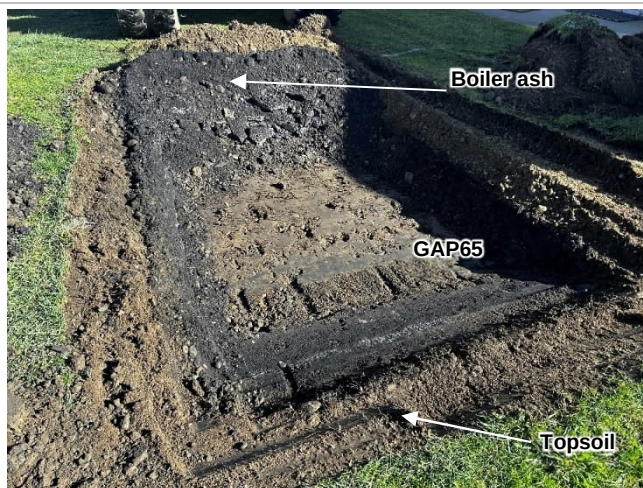
Photograph 11. View of TP18 showing boiler ash layer
