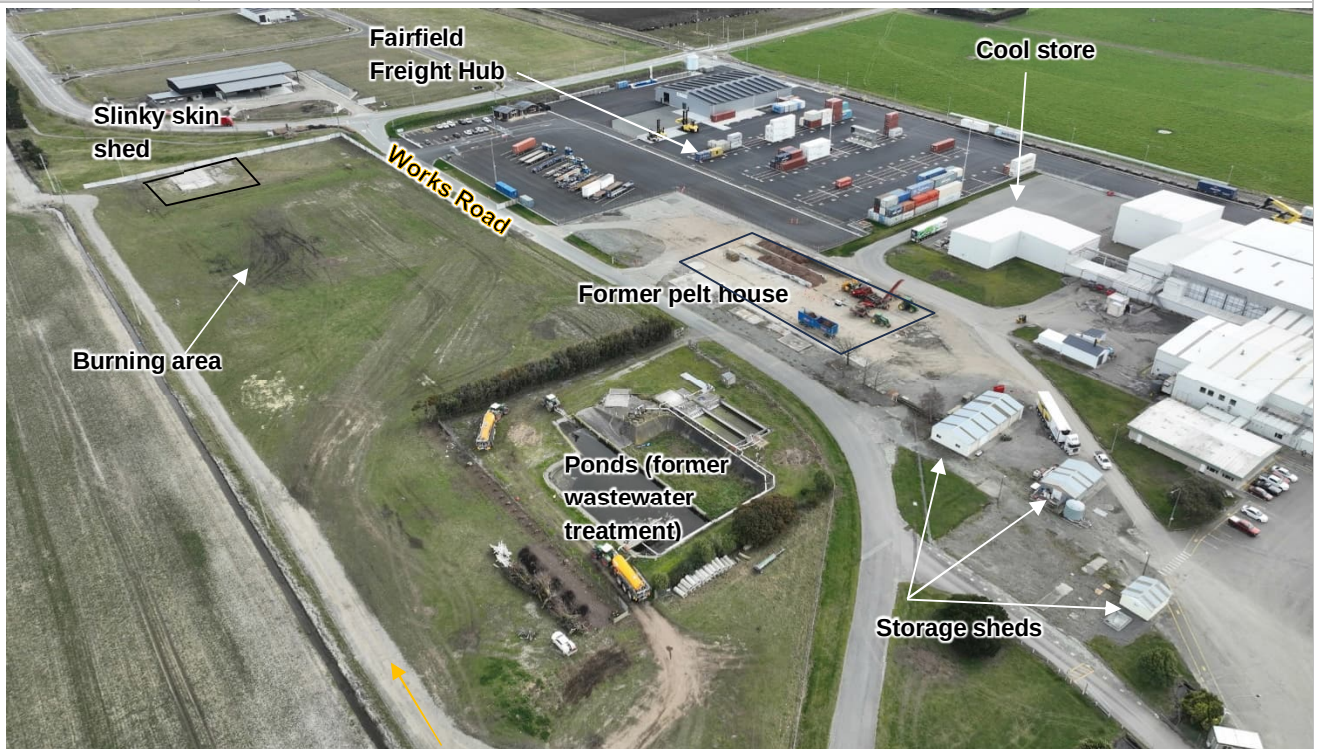
Photograph 5. Drone image showing the central third (flown by Tarbotton Land & Civil, August 2024).
