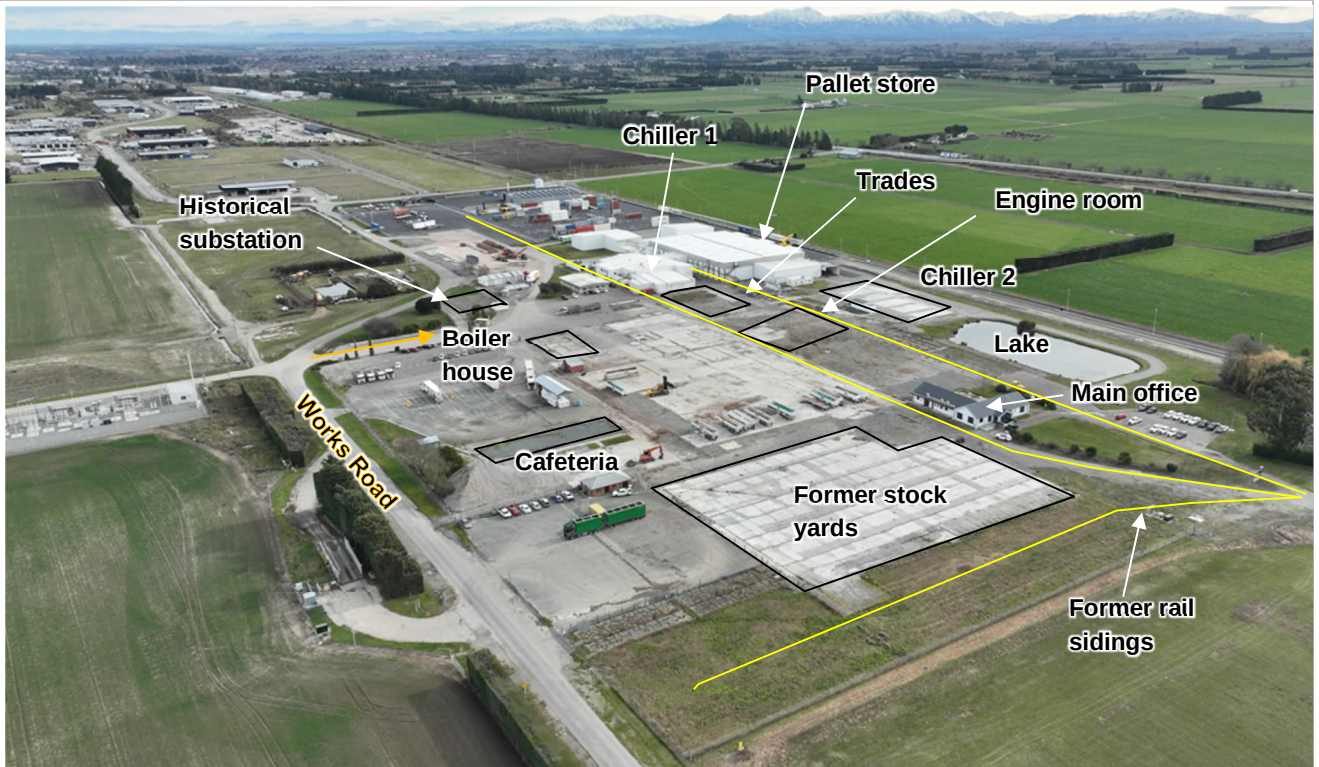
Photograph 4. Drone image showing the central portion of the site (flown by Tarbotton Land & Civil, August 2024).
