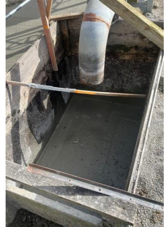
Newly concreted floor
