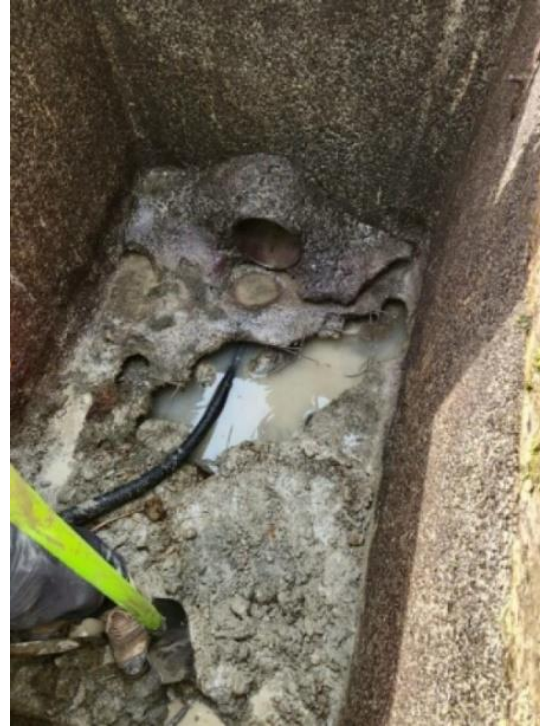
Damaged floor of offtake chamber
