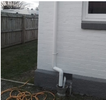
A downpipe illegally discharging into a wastewater gully trap.
