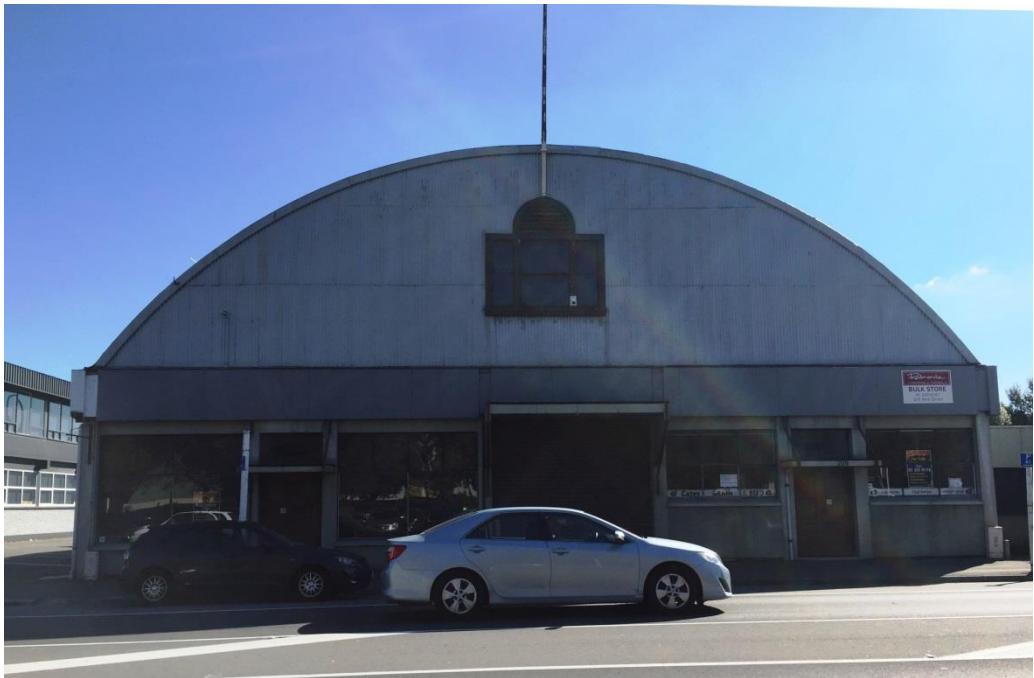
Figure 1. Eastern elevation, Cates Grain Store, Ashburton (List no. 1807), 17 April 2019, C. Whybrew (Heritage New Zealand Pouhere Taonga)
