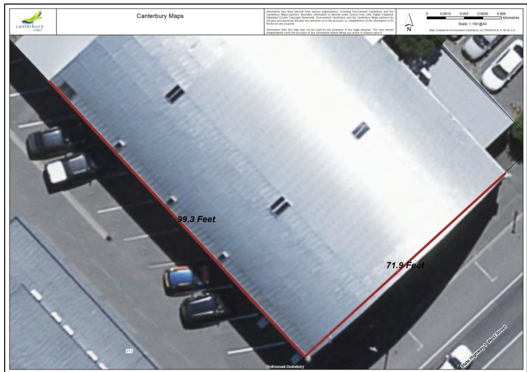
Figure 4. Latest aerial imagery from Canterbury Maps showing approximate dimensions of original building, Cates Grain Store (in feet).
