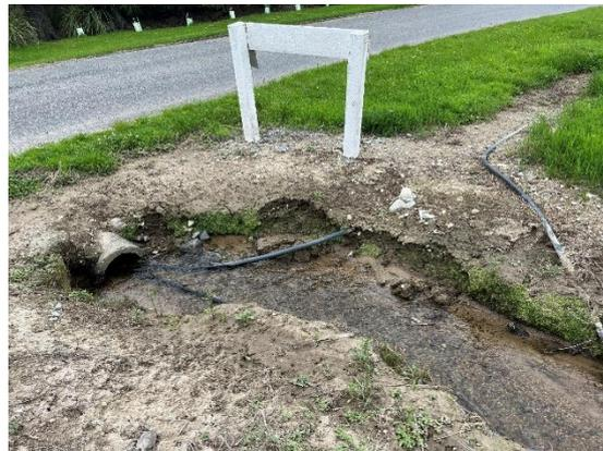
*Figure 5. Alford Forest stock water channel entering culvert as it crosses the road at Site 4. Exposed banks indicate damage from unprotected riparian margins.*
