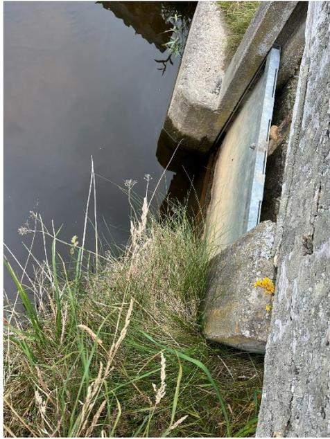
Figure 6 (Right). Weir plate that allows flow diversion to be adjusted. Permanently lowering the plate would stop the diversion but would need to be made permanent to prevent future unauthorised takes from Limestone Creek.
