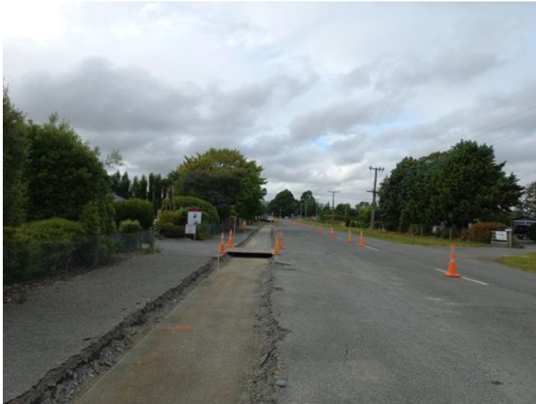
Albert St, Ashburton – prepared for kerb and channel
