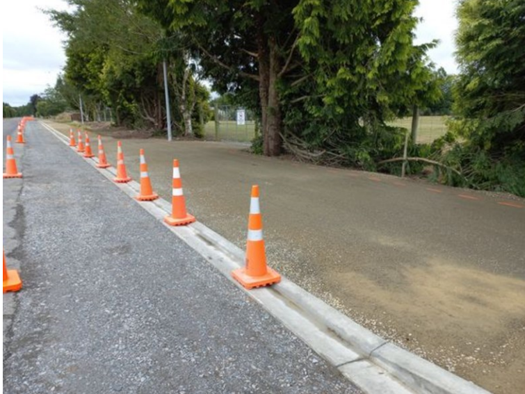
Dolma St, Methven footpath preparing for seal
