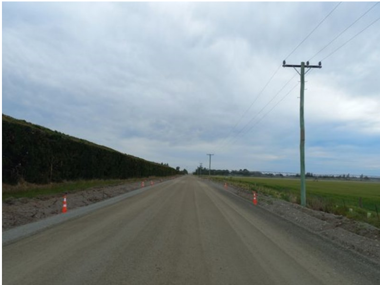
Tinwald Westerfield Mayfield Rd prior to sealing
