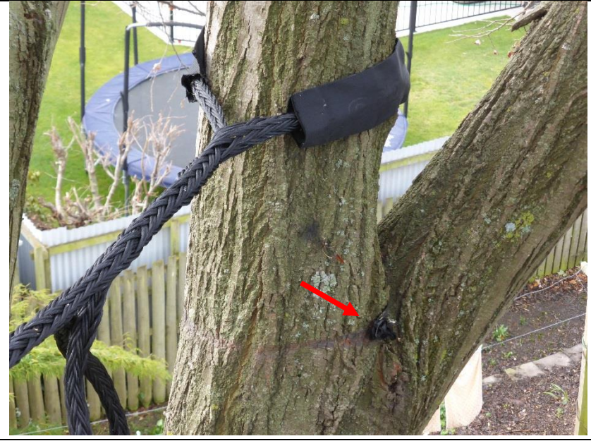
Photo 5: Previously failed cobra system partially included at the point of attachment.
