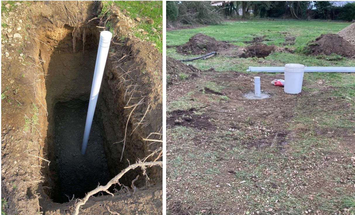
Figure 2. Test Pit 1 with Piezometer installed.
