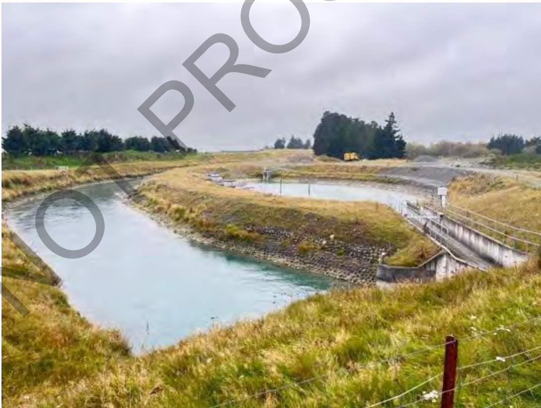
Figure 35, Ashburton South Branch siphon and settling pond on the RDR
