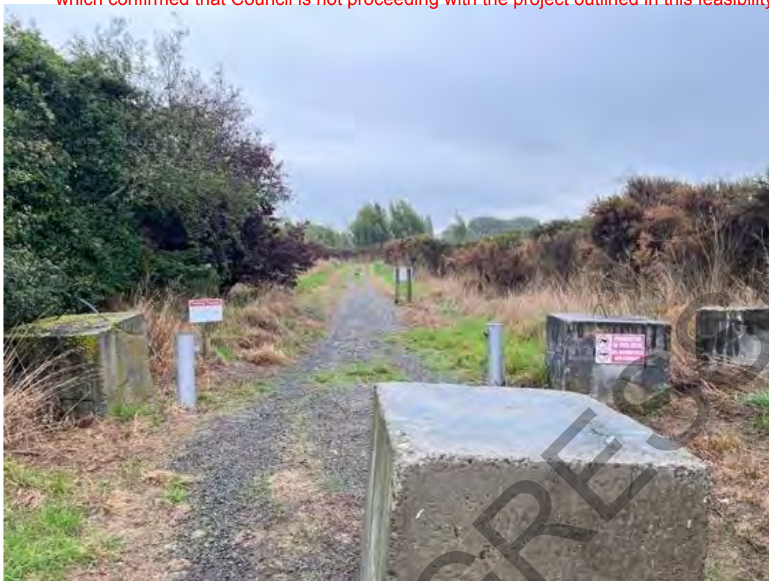
Figure 53, Squeeze barriers at Cochranes Road
