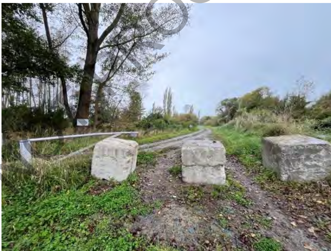
Figure 52, Squeeze barriers at Milton Road south
