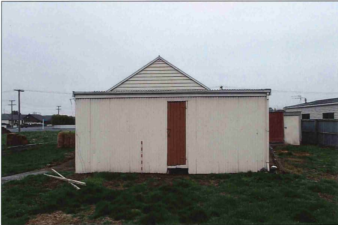
Figure 36. Shed 3, northwest elevation of the lean-to. Note the ledged and braced door made from narrow (85 mm) boards.
