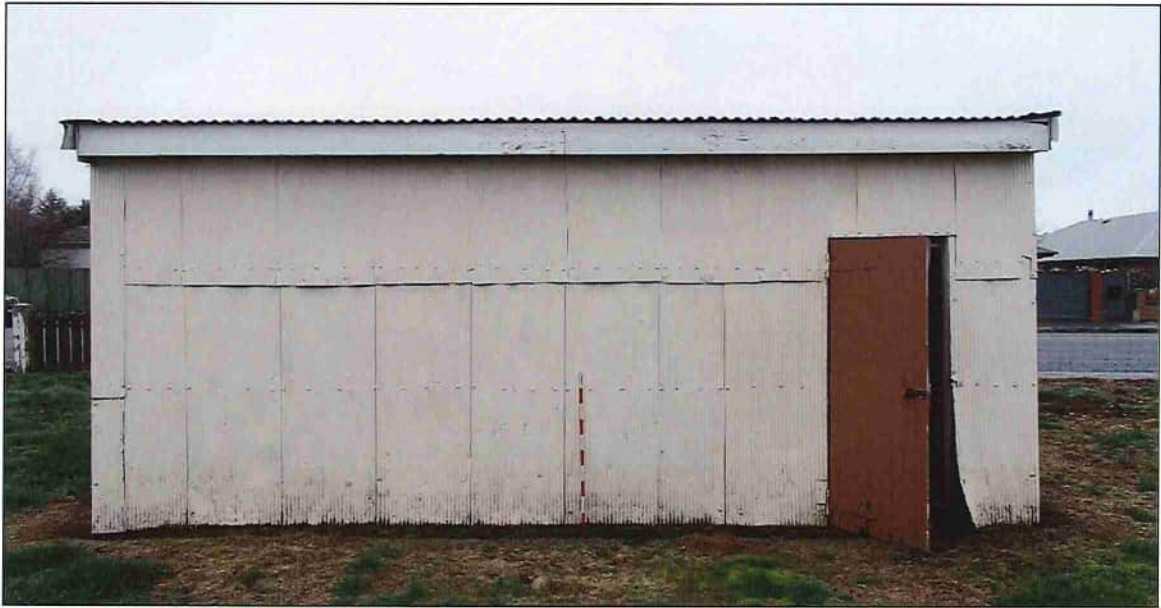
Figure 30. (Above) Shed 2, southwest elevation. Note the ledged and braced door. Scale = 10 cm increments.
