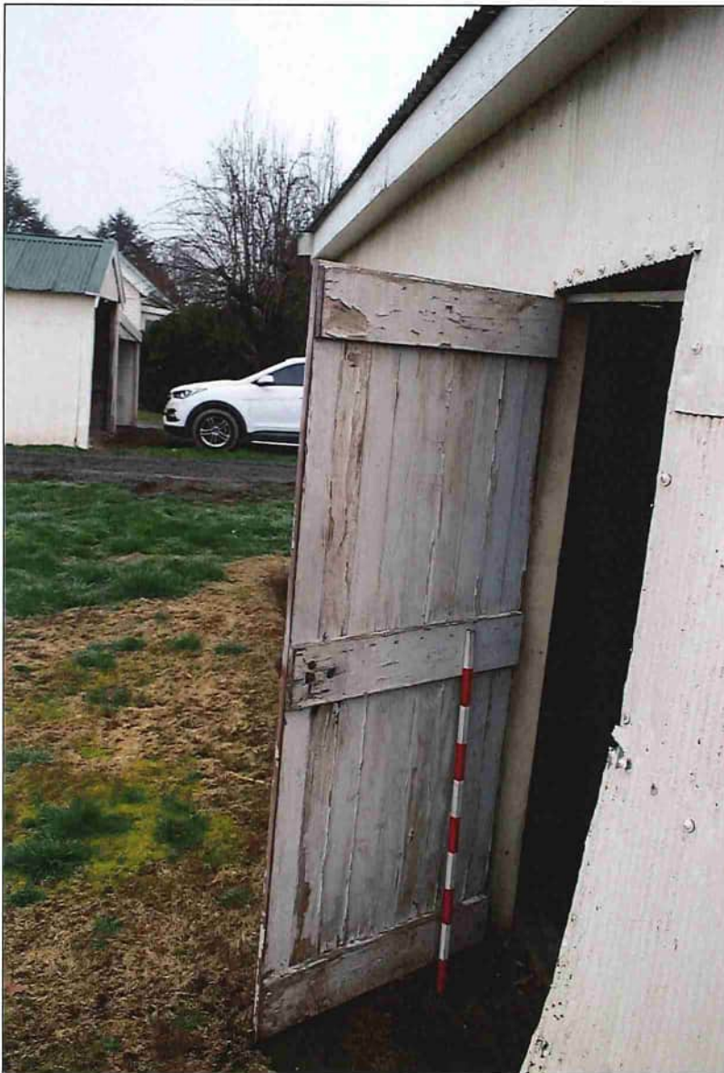
Figure 30. (Above) Shed 2, southwest elevation. Note the ledged and braced door. Scale = 10 cm increments.
