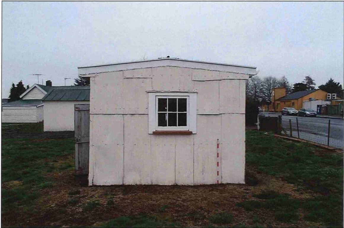
Figure 32. Shed 2, southeast elevation. Note the casement window. Scale = 10 cm increments.
