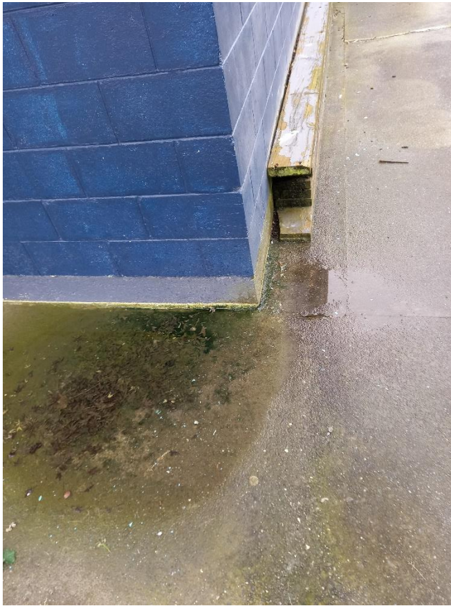
View of south-east corner of building, surface water ponding and external slab cracked with level differences across the crack, all evidence of past settlement of the foundation.
