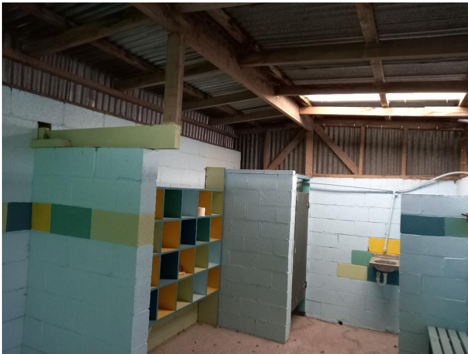
Internal of female changing rooms showing hollow block partition walls. Note right hand wall shows signs of past lateral and horizontal movement.
