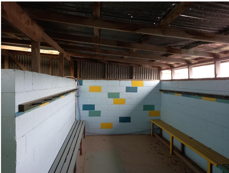
View within the same female changing room looking toward the northern external wall showing the same 35mm open gap at the top where it joins the original structure to the left.
