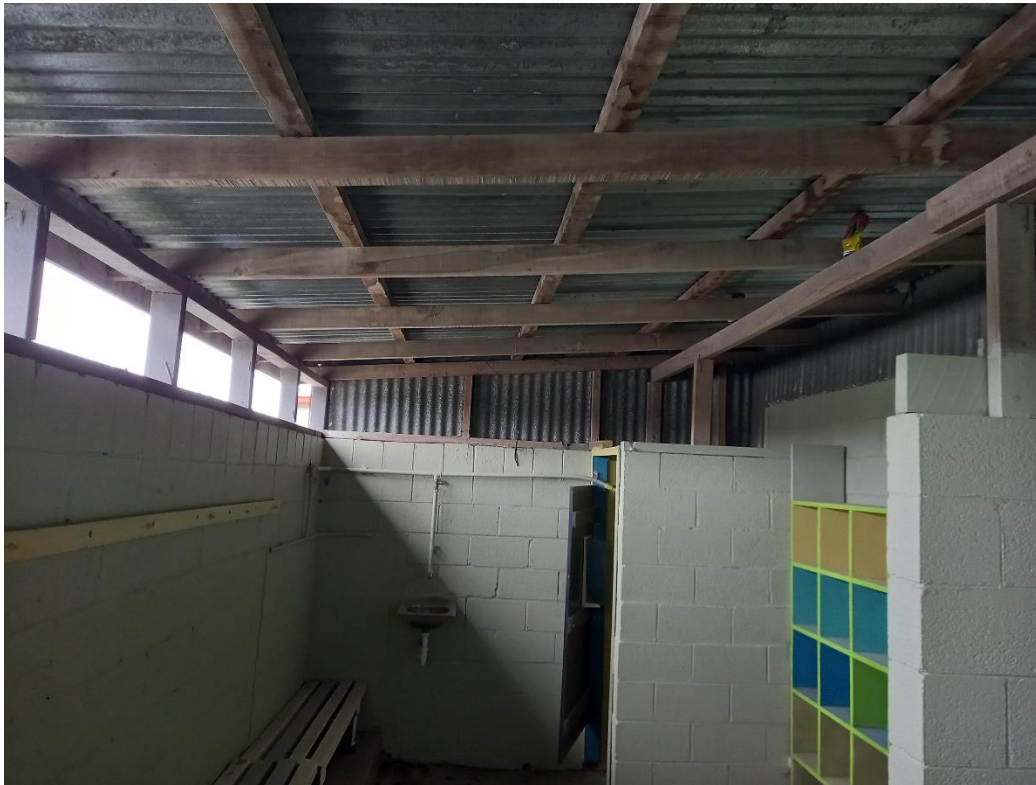
Internal of Male changing room showing sawtooth crack filled on north wall and short internal hollow block partition walls.
