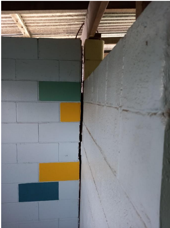
View of south external wall internally within female changing room showing 35mm open gap at top of wall where the eastern elevation wall foundation has appeared to have settled causing the connected south wall to rotate.
