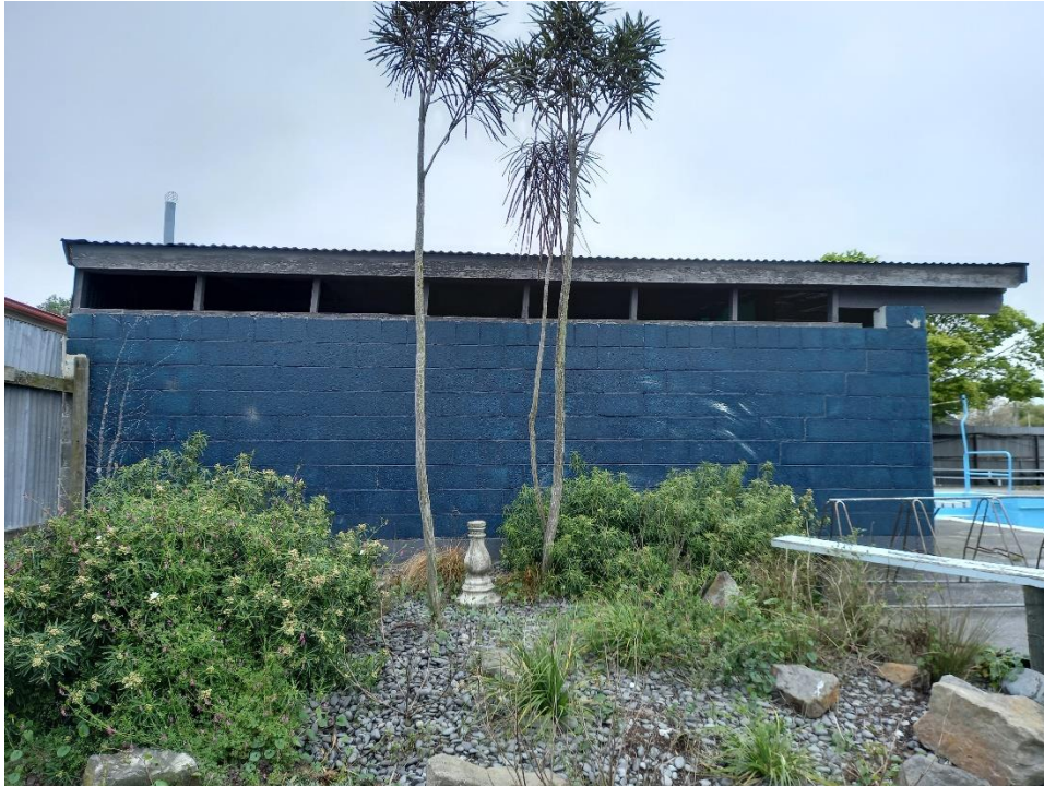
West Elevation showing filled saw-tooth cracking at south end and short timber jack studs leaning noticeably to the south.
