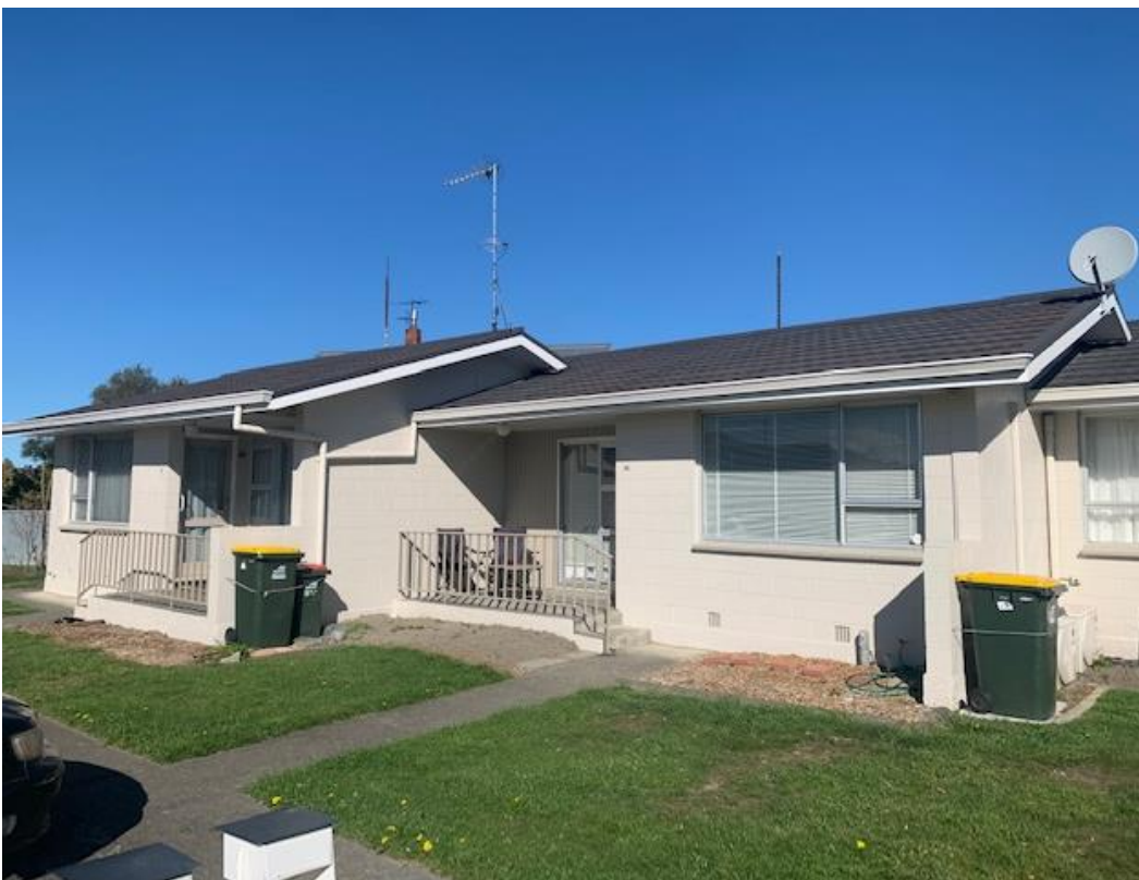
Units 5, 6 and 7 Elizabeth St Ashburton received a full exterior repaint 1 years ago
