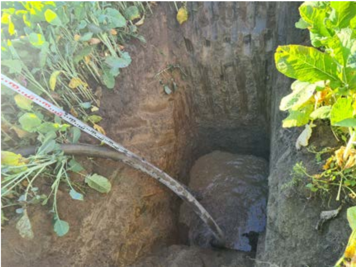
Photo – Soakage Test Pit 6
