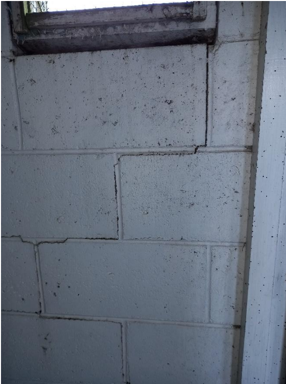
View of Male Toilet cubicle south wall and cracking to the hollow blockwall joints, symptomatic of past seismic movement.
