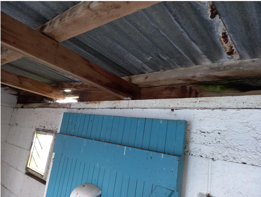
View internally of south wall in the male changing room showing end of one rafter missing and rotten and borer damage top plate.
