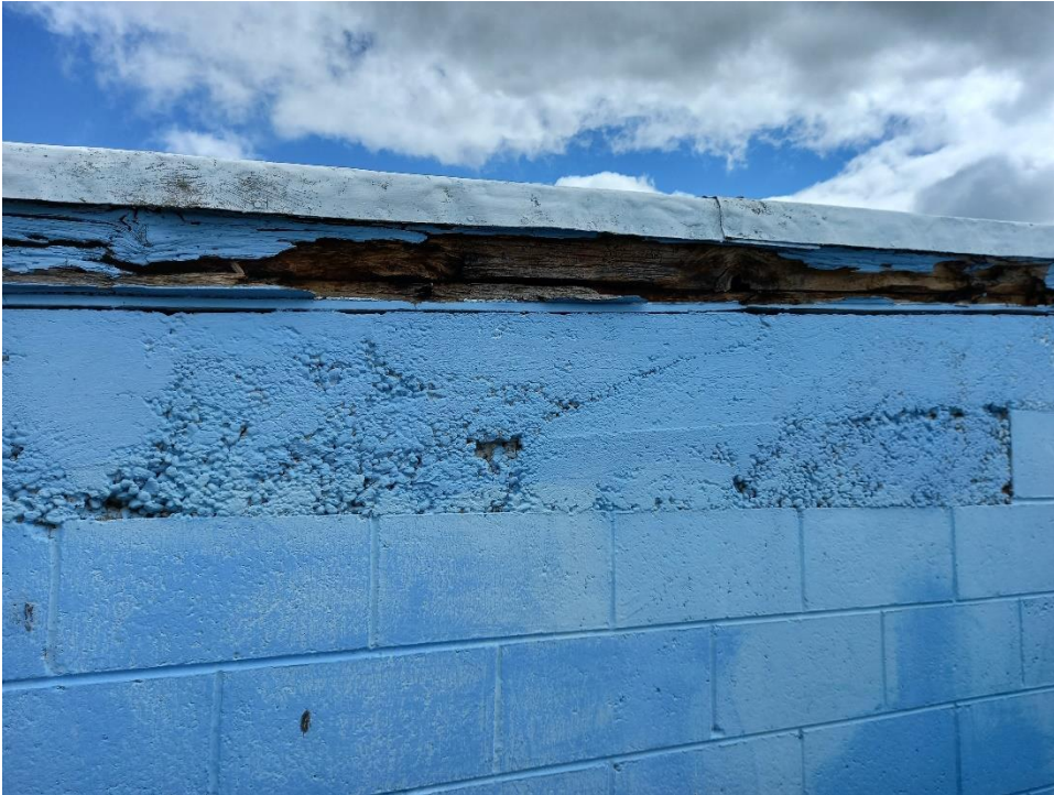
East End view of roof barge board totally rotten through with holes to the inside.
