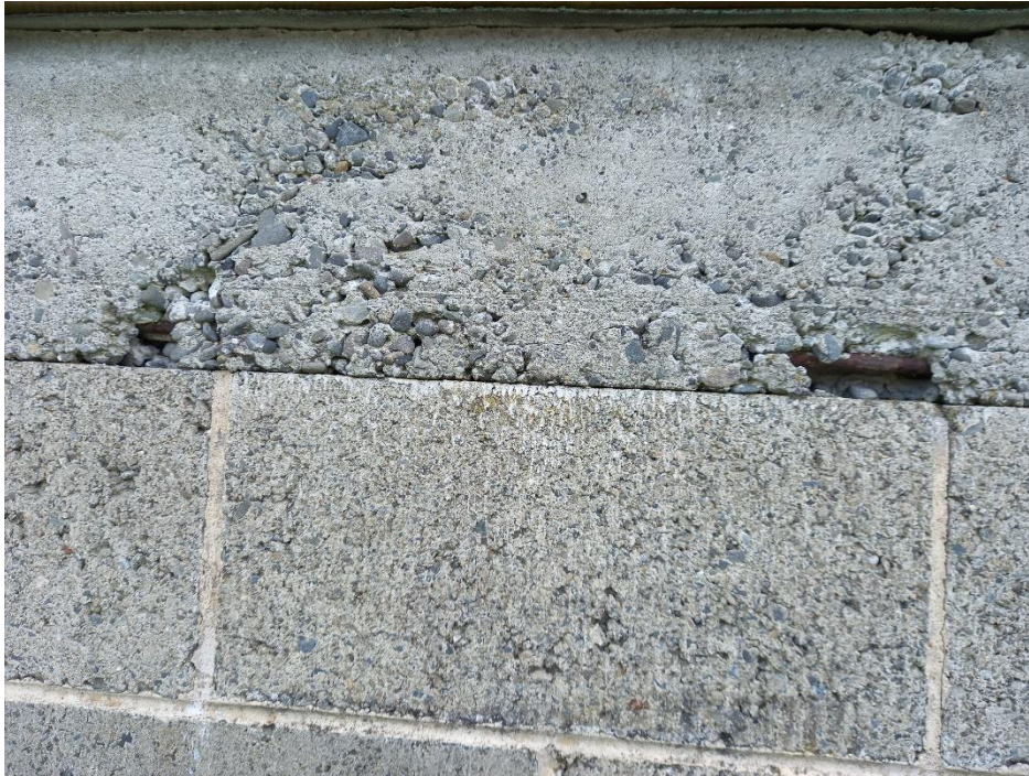
South Elevation concrete bond-beam showing poor original concrete compaction and low cover leading to reinforcement corrosion and spalling of concrete.
