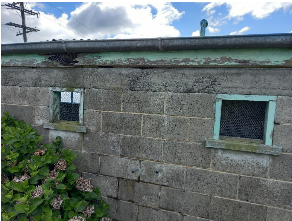
South Elevation above toilet windows showing rotten fascia board open to rain ingress and cracks below the left hand window in the joints.
