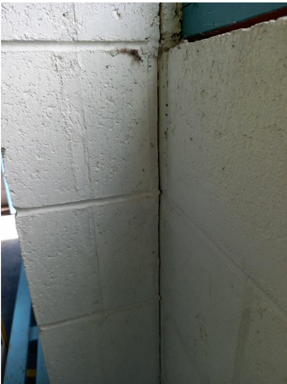
View of detachment of another block pier from the blockwall within the female changing room on the north wall.
