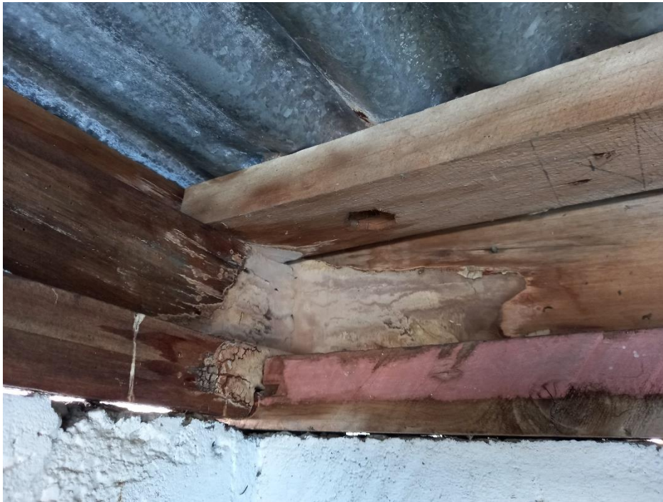
View of the south-east corner of the female changing room showing white fungus rot to all timber members and daylight under bottom plate.
