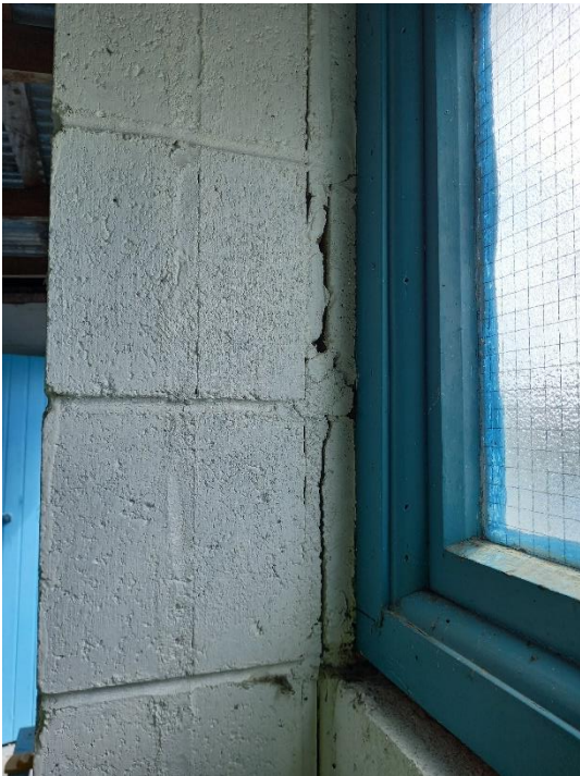
View of detachment of female changing room blockwork pier from north external wall, most likely during past seismic event.
