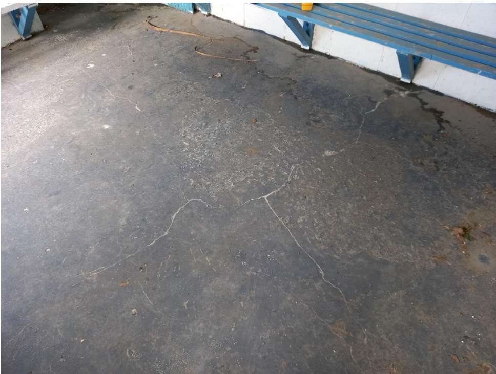
View of male changing room floor slab showing past floor slab cracking that has been filled in the past.
