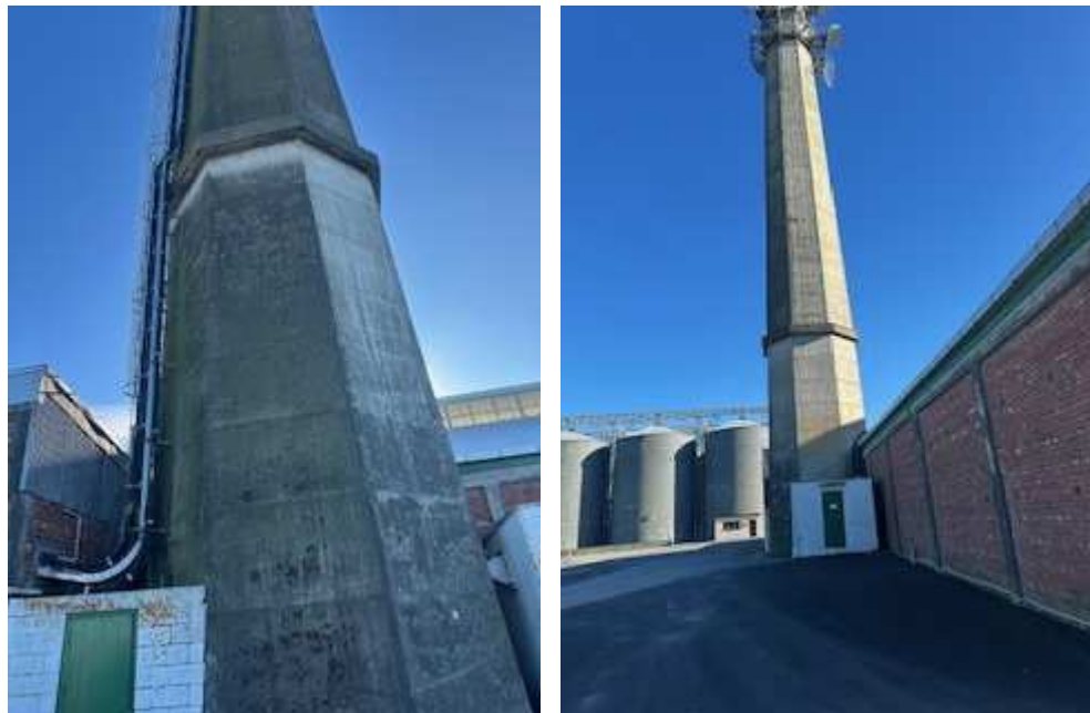
Photo 6. Photo of chimney – at left shows the collar at circa 7-8m high – that is the partial demolition height proposed.
