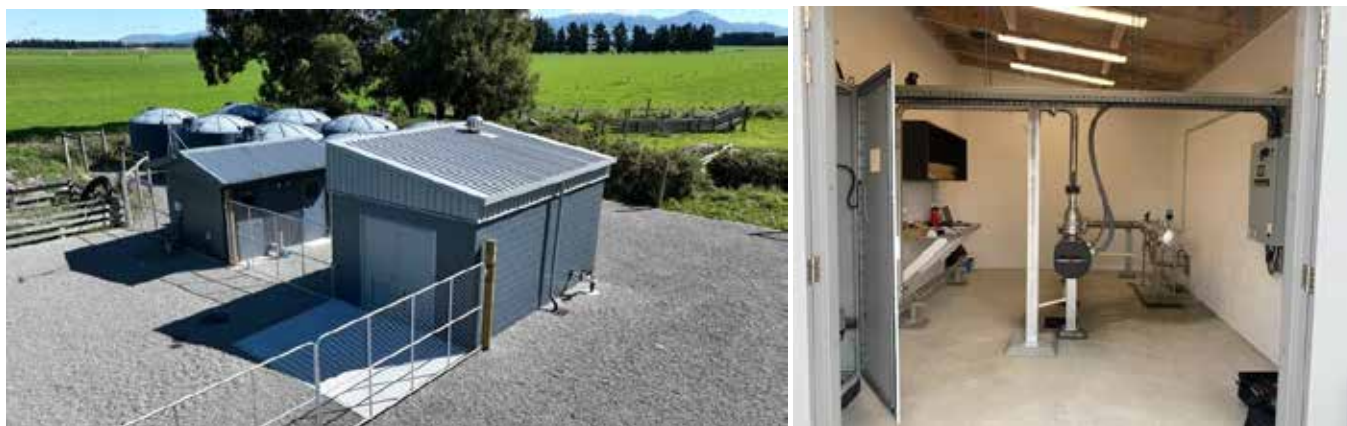
Mayfield drinking water plant (left), and UV equipment (right).
