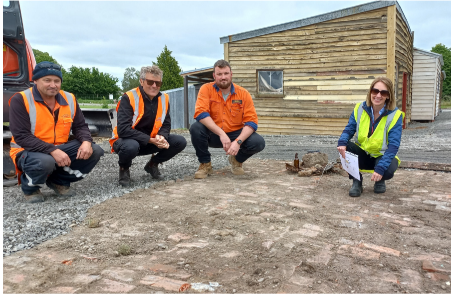
Council staff and contractors inspect the brick floor.
