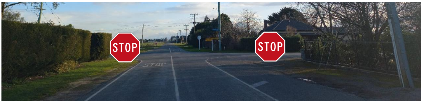
Longbeach Rd / Boundary Rd (East Approach) – Upgrade to large 1200mm stop signs and white background 200mm stop ahead (gated).
