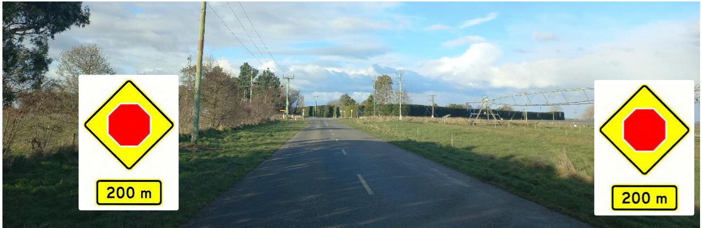
Poplar Rd / Coldstream Rd (East Approach) – Change to Stop Control. Upgrade to large 1200mm stop signs and white background 200mm stop ahead (gated). Poor visibility to the right.
