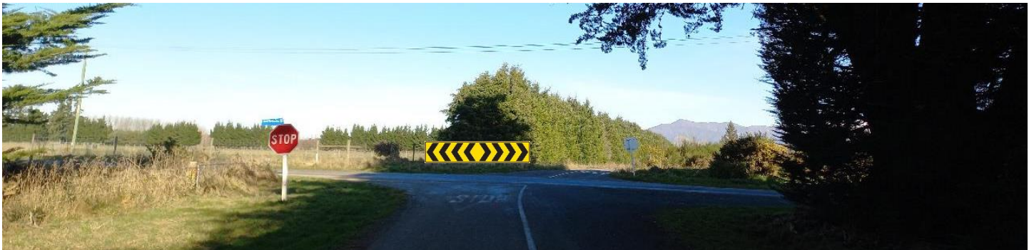
Jones Road / Hinds Arundel Road – Re-locate 1x Give Way advanced warning signs from Ealing Montalto/ Hinds Arundel after upgrade. Install PW 68 T-Intersection Chevron on opposite side of intersection.
