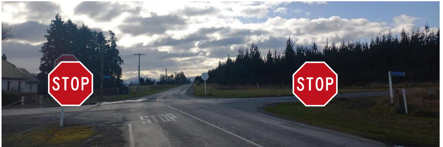
Ealing Montalto Road / Trevors Road (South Approach) – Upgrade to large 1200mm stop signs and white background 200mm stop ahead (gated).
