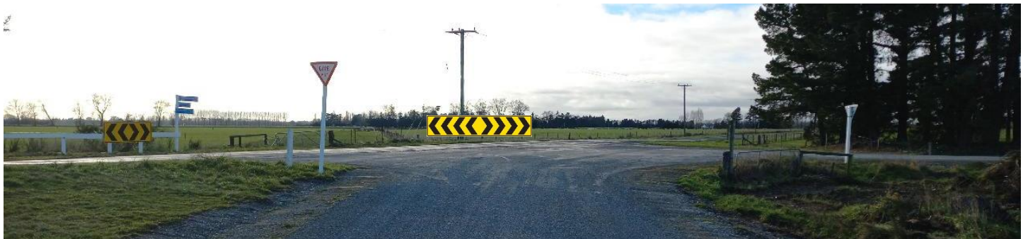
Tinwald Westerfield Mayfield Road / Rushford Road – Install PW 68 T-Intersection Chevron
