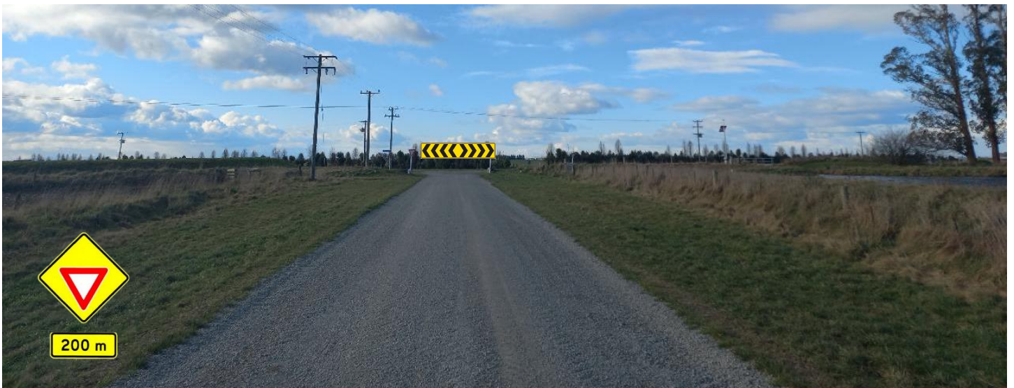
Jones Road / Hinds Arundel Road – Re-locate 1x Give Way advanced warning signs from Ealing Montalto/ Hinds Arundel after upgrade. Install PW 68 T-Intersection Chevron on opposite side of intersection.
