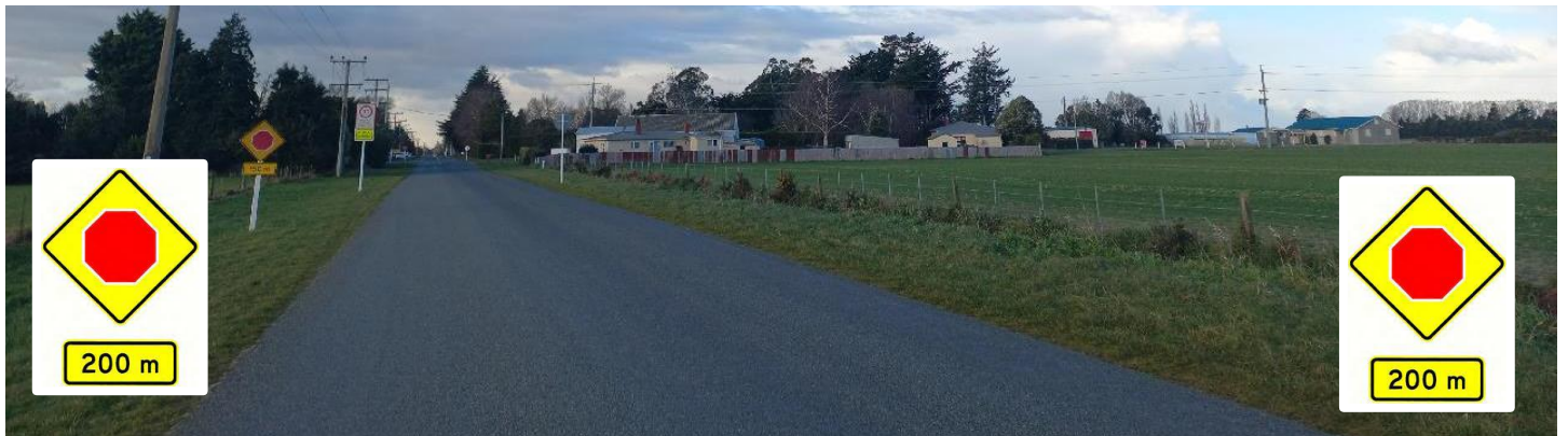
Longbeach Rd / Boundary Rd (East Approach) – Upgrade to large 1200mm stop signs and white background 200mm stop ahead (gated).
