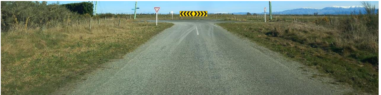
ARG / McKenzies Road – Install PW 68 T-Intersection Chevron
