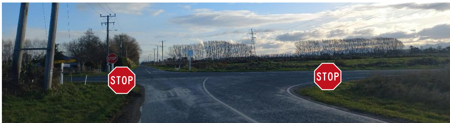
Fords Rd / Boundary Rd (East Approach) – Upgrade to large 1200mm stop signs and white background 200mm stop ahead (gated). Avenue effect due to power lines and trees.
