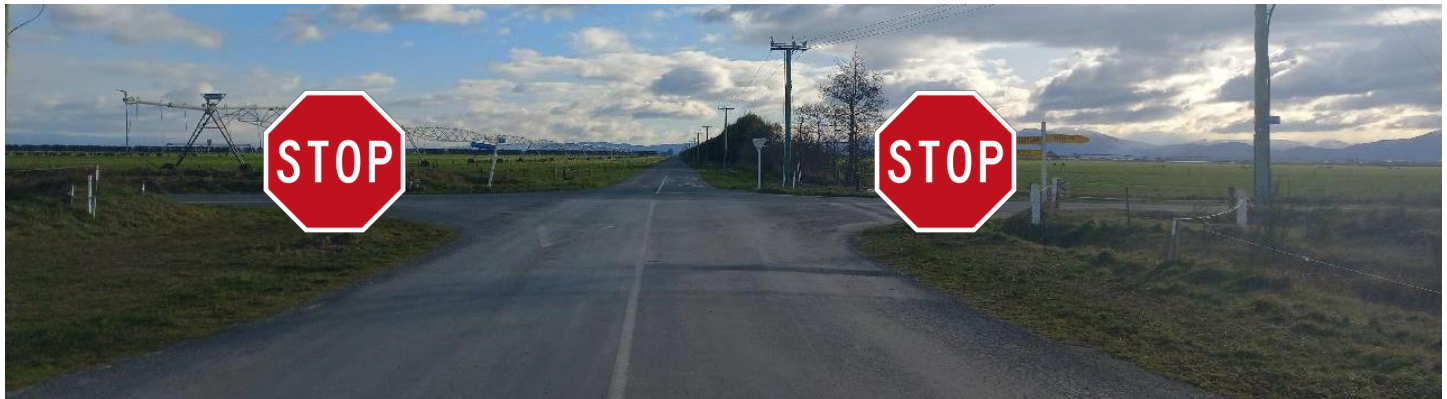
Poplar Rd / Coldstream Rd (East Approach) – Change to Stop Control. Upgrade to large 1200mm stop signs and white background 200mm stop ahead (gated). Poor visibility to the right.
