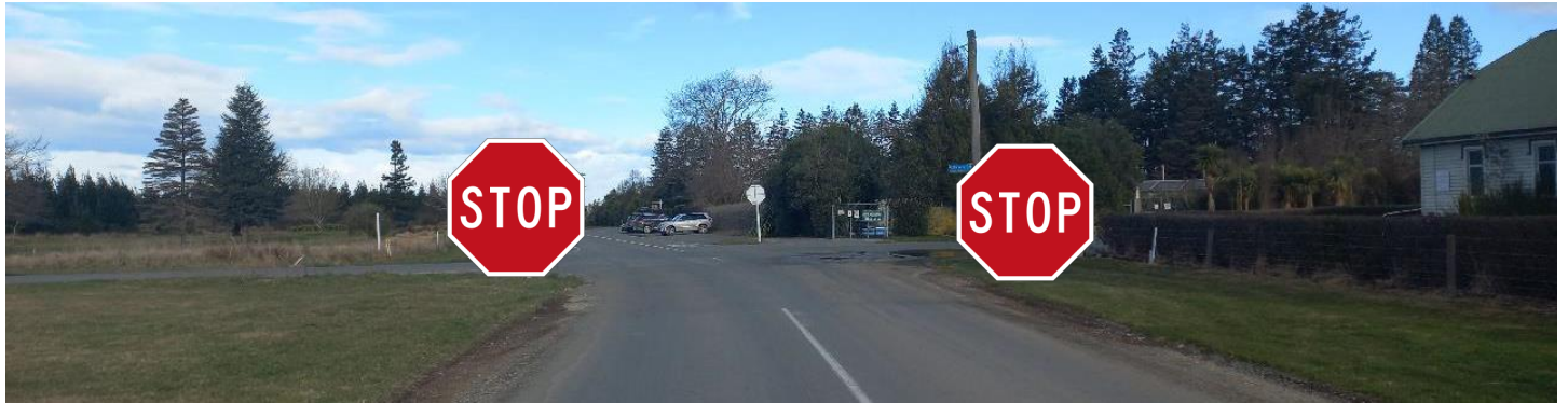
Ealing Montalto Road / Trevors Road (North Approach) – Upgrade to large 1200mm stop signs and white background 200mm stop ahead (gated).
