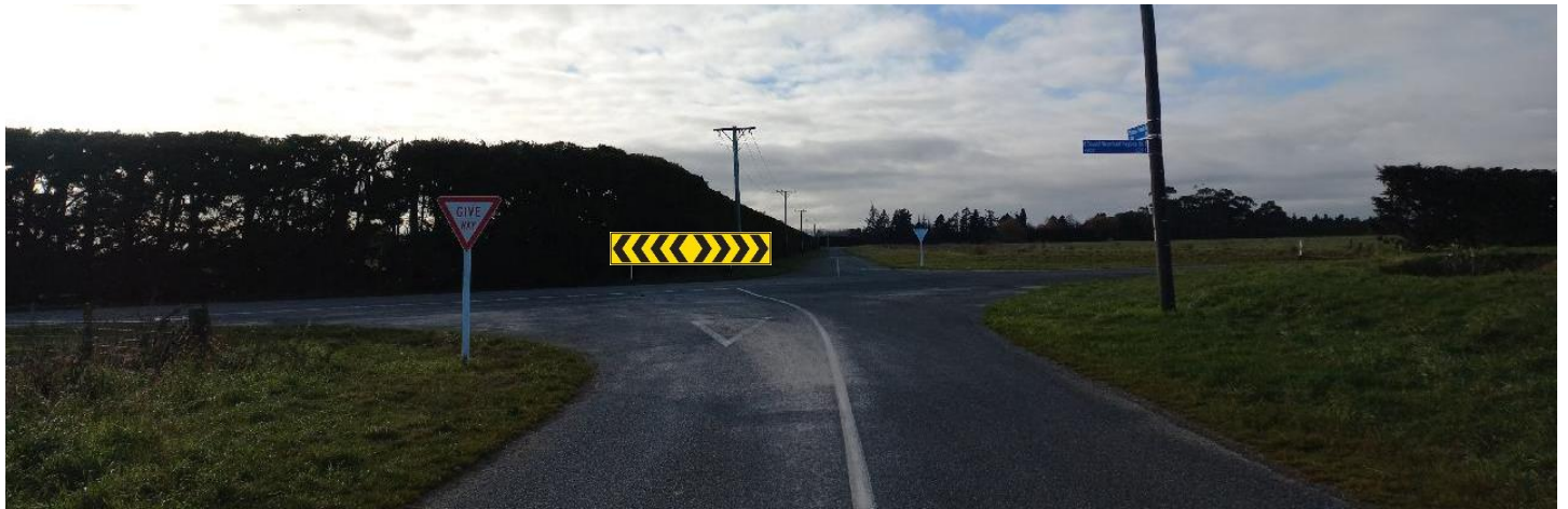
Tinwald Westerfield Mayfield Road / Rushford Road – Install PW 68 T-Intersection Chevron
