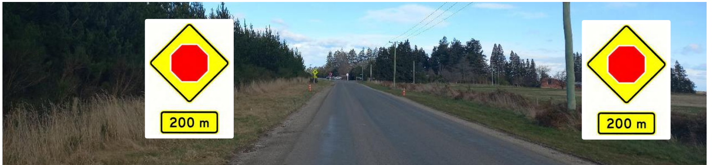
Ealing Montalto Road / Trevors Road (South Approach) – Upgrade to large 1200mm stop signs and white background 200mm stop ahead (gated).
