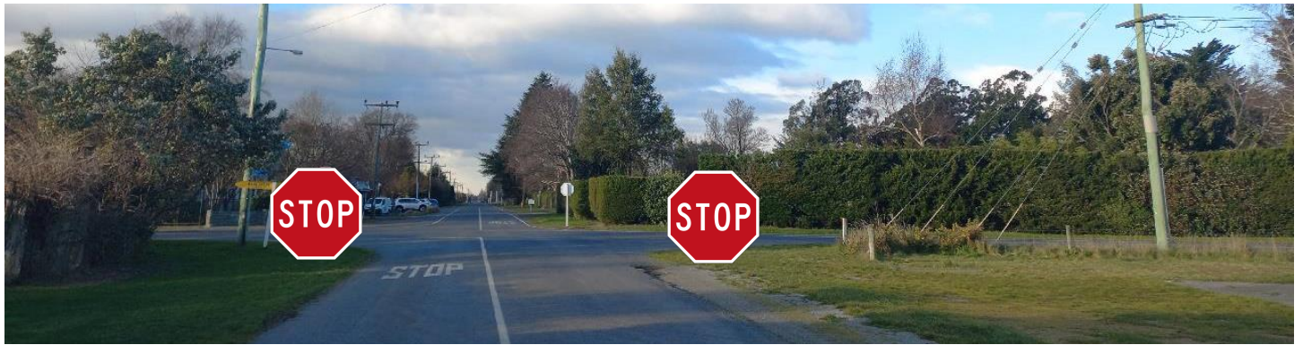
Longbeach Rd / Boundary Rd (West Approach) – Upgrade to large 1200mm stop signs and white background 200mm stop ahead (gated).
