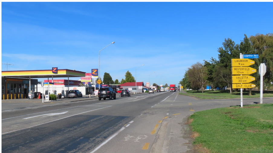
Traffic signals will be installed at the intersection of SH1/Lagmhor Road/ Agnes Street to create regular gaps for side street traffic.
