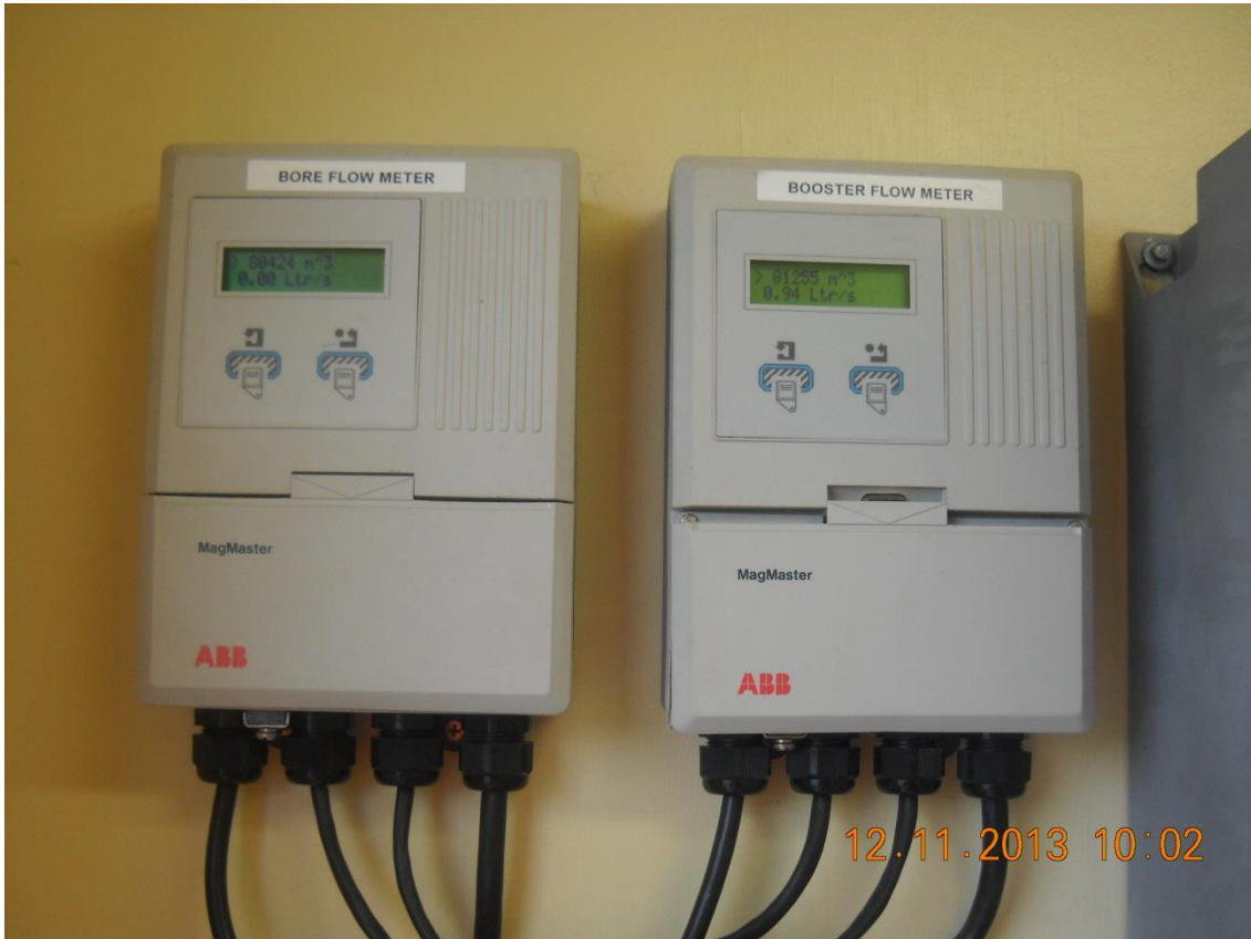
Photo 5: Flow meter equipment
