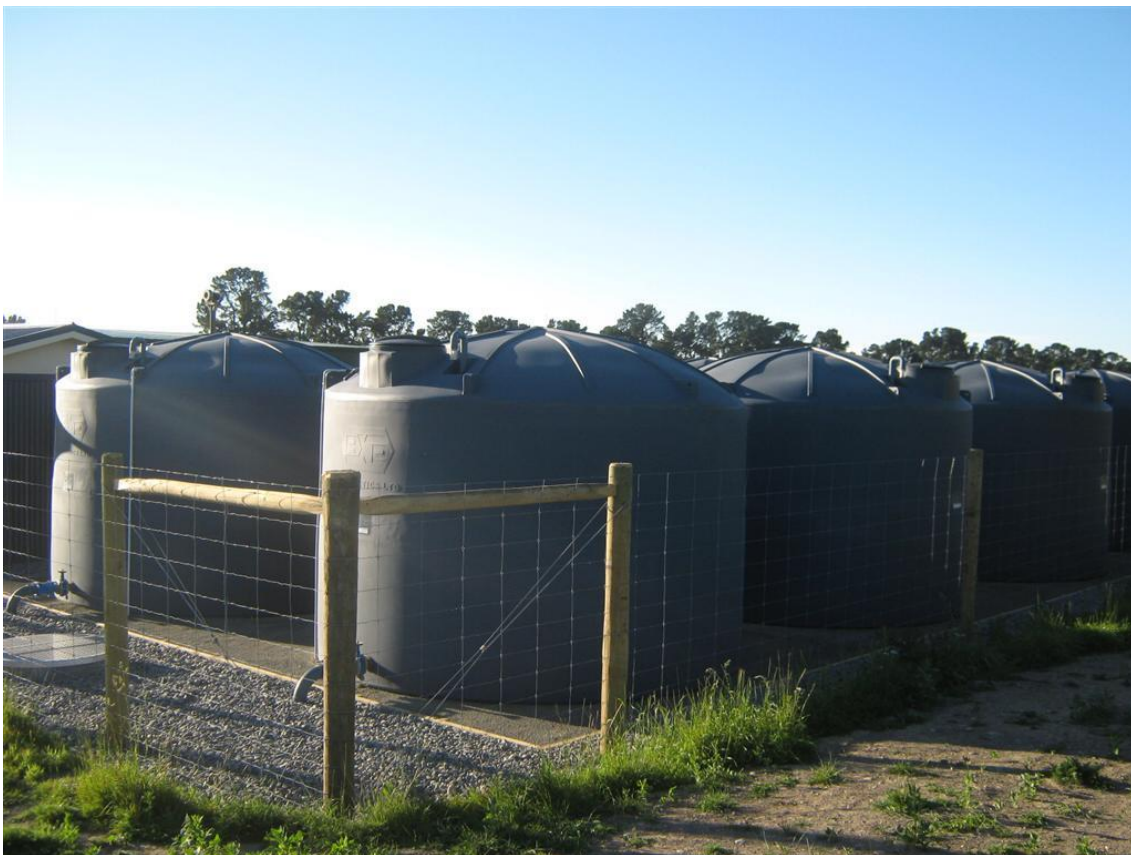
Photo 6: Eight 33m 3 supply reservoirs in fenced compound
