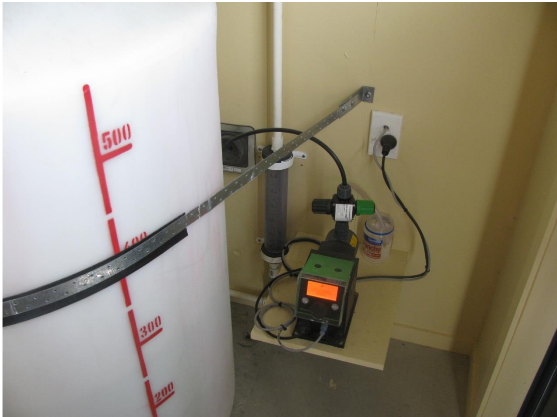
Photo 4: Chlorine tank, scale tube, and dosing pump
