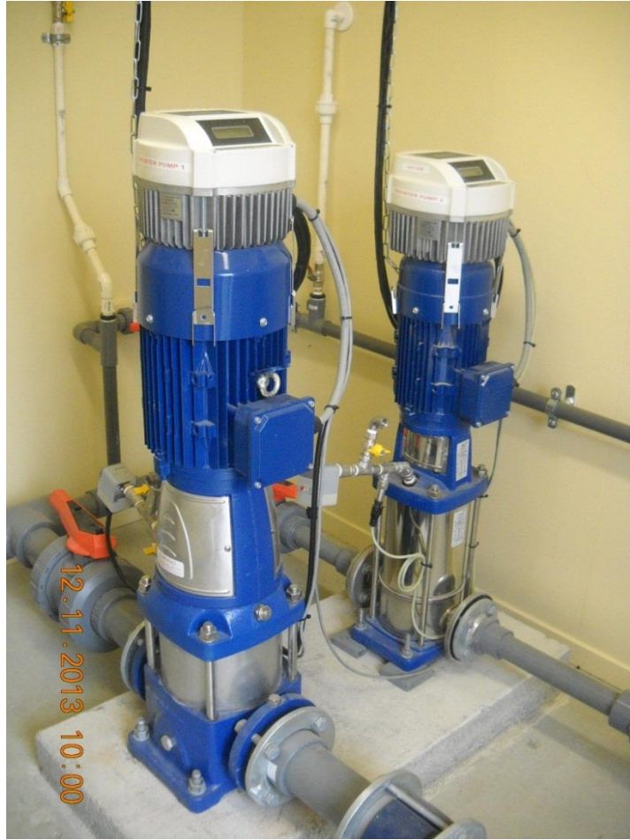
Photo 7: Water distribution (booster) pumps
