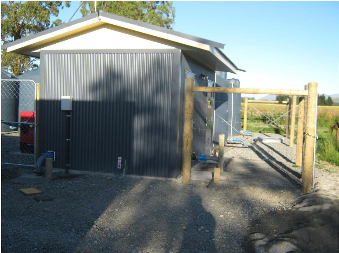
Photo 3: Mayfield treatment plant and pump station building
