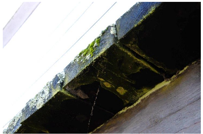
Figure 91: Lichen and moss growth to the timber deck of the bridge.
