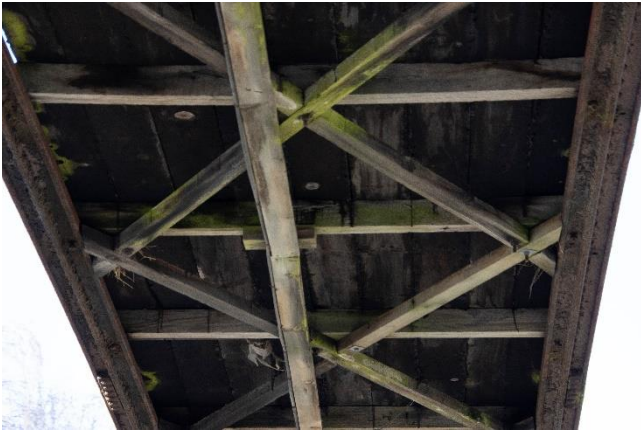
Figure 82: Algae growth to the underside of the bridge.
