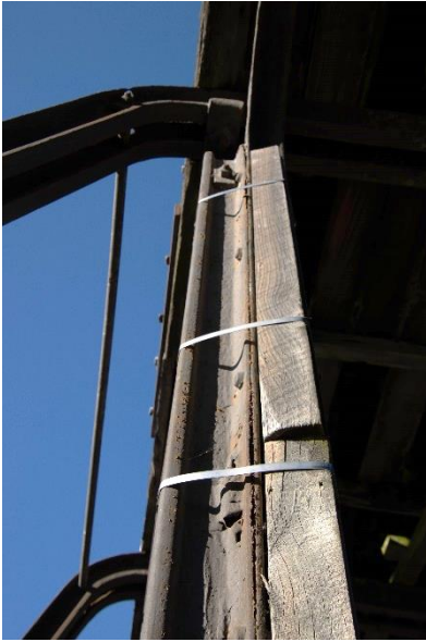
Figure 94: Timber strengthening to metal support, with metal cable ties.
