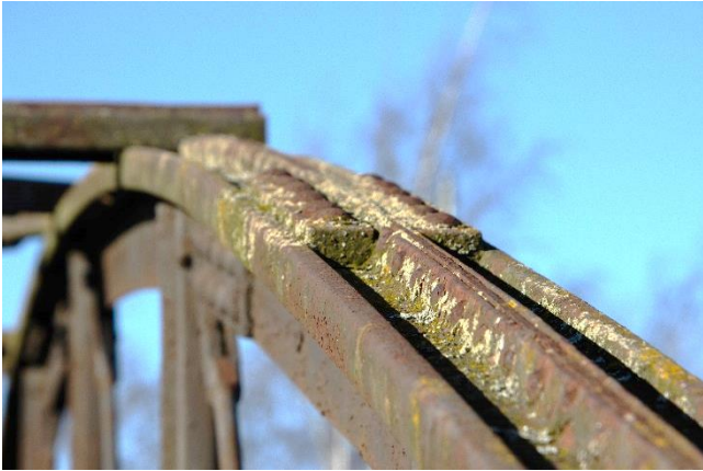
Figure 88: Lichen growth to the ferrous elements of the bridge.
