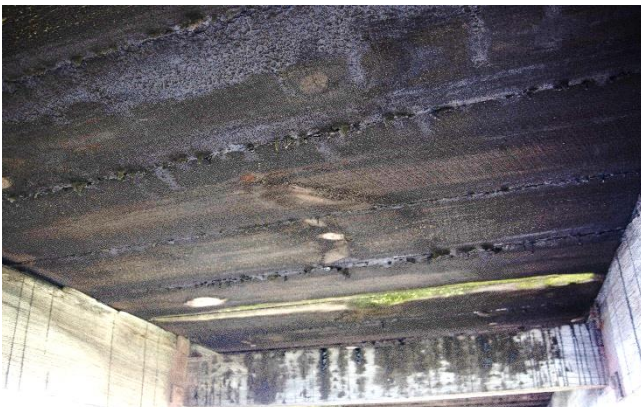
Figure 84: Algae growth to the underside of the bridge.
