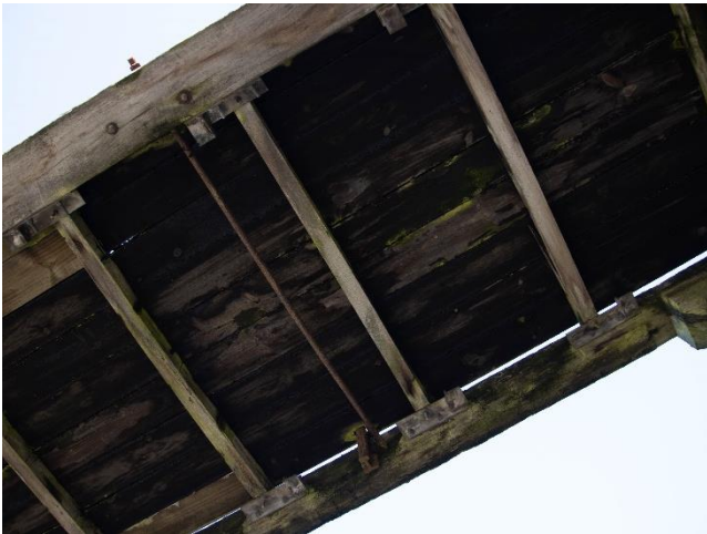
Figure 70: Metal tie rod to the underside of the timber bridge structure.
