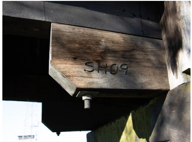
Figure 71: One of many timber inserts visible in the bridge structure, marked with 'SH09'.
