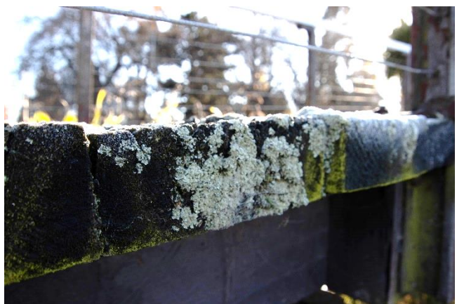
Figure 87: Lichen growth to the bridge deck.
