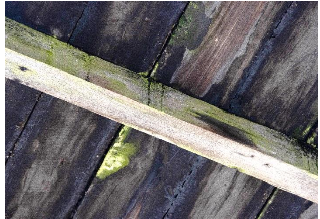
Figure 83: Algae growth to the underside of the bridge.
