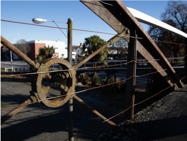
Figure 52: The diagonal tierods with central circular tensile connector in one of the trusses of the bridge.
