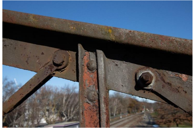
Figure 73: Corrosion to the cast iron elements of the bridge span is visible to the entire structure.
