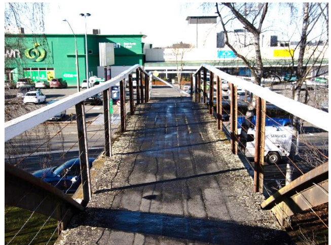
Figure 61: The timber deck structure with asphalt surface.
