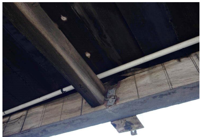
Figure 81: Runoff from the bituminous layer added to the deck surface when installed.
