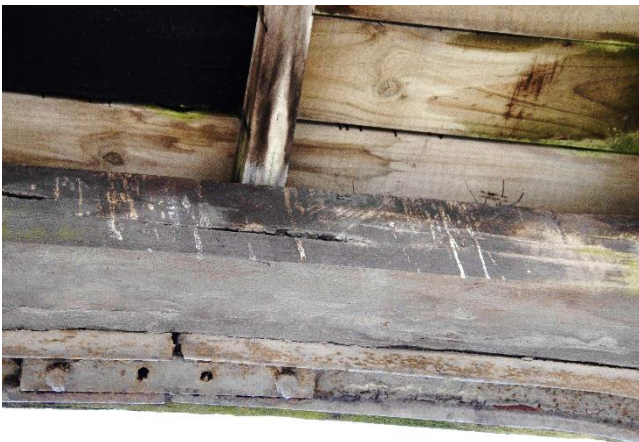
Figure 78: Bird droppings to the underside of the bridge structure.
