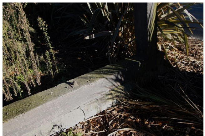
Figure 77: Cracks to the concrete foundations which sit below the timber trusses underneath the ramped section of the footbridge.
