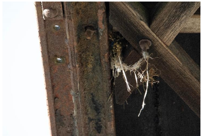
Figure 79: One of multiple bird nests in the structure.
