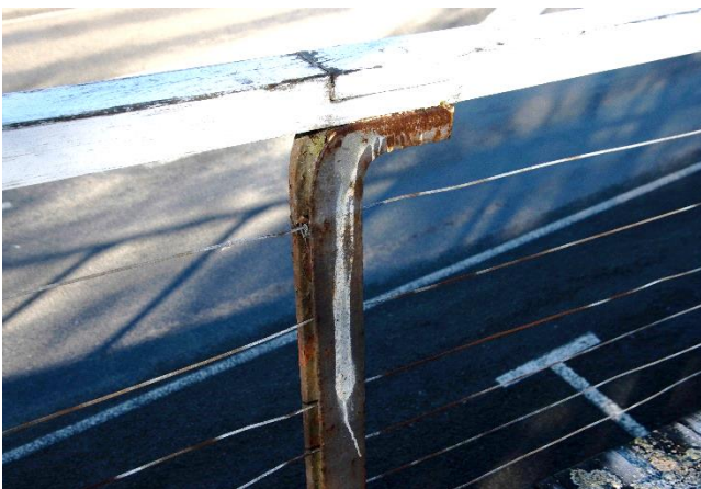
Figure 80: Paint running down the metal balusters on the footbridge from when the handrail was painted.
