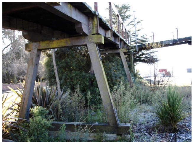
Figure 67: Timber supports on concrete foundations to the ramped footbridges to either side of the main bridge span.
