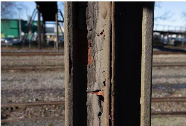
Figure 74: Corrosion to the metal supports across the entire structure is visible under a layer of flaking paint.
