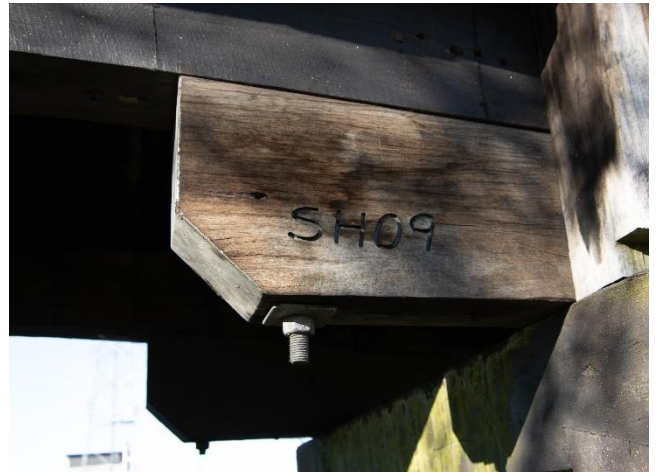
Figure 97: Timber inserts, some marked with 'SH09', inserted into the structure.
