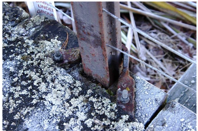
Figure 75: Corrosion to the metal handrail balusters and brackets is evident across the entire structure.
