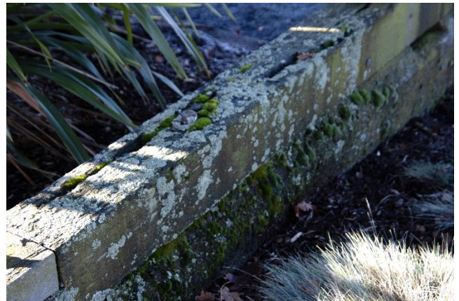
Figure 93: Lichen and moss growth to the timber supports of the bridge.
