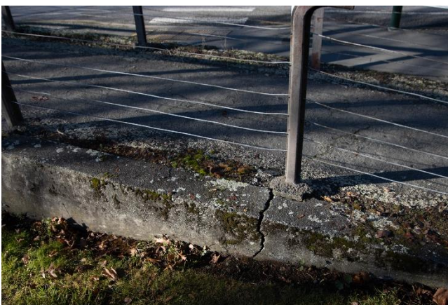
Figure 76: Cracks to the concrete ramp base on the eastern side of the bridge.
