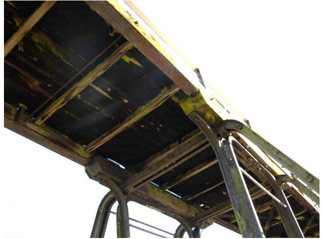
Figure 69: Where the metal supports meet the timber structure of the bridge.
