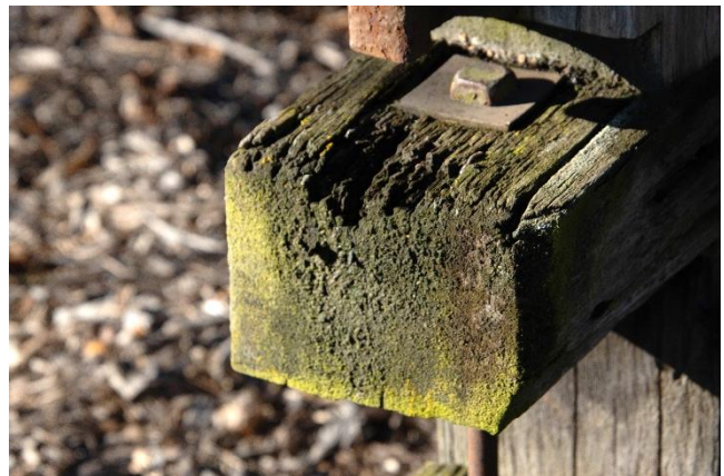
Figure 85: Algae growth to the underside of the bridge.
