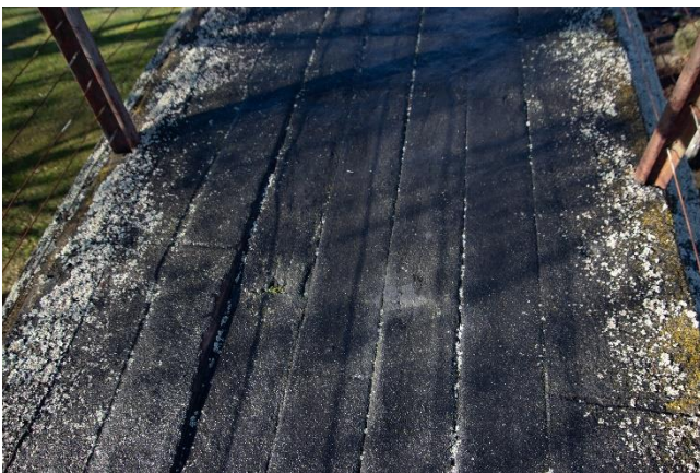
Figure 90: Lichen growth to the timber deck of the bridge.
