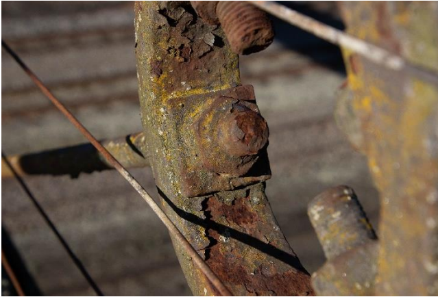
Figure 72: Corrosion to the cast iron elements of the bridge span is visible to the entire structure.
