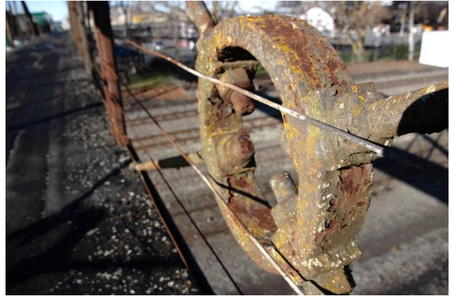
Figure 89: Lichen growth to the ferrous elements of the bridge.
