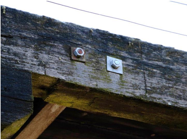
Figure 96: Different bolts are visible haphazardly installed across the structure.
