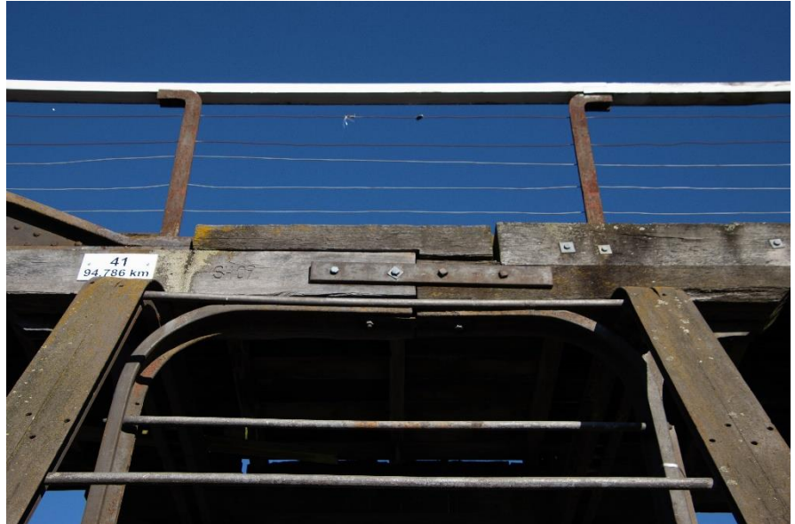
Figure 95: Previous repairs where various timber inserts (some marked with 'SH09') have been spliced into the existing structure and screwed into place.
