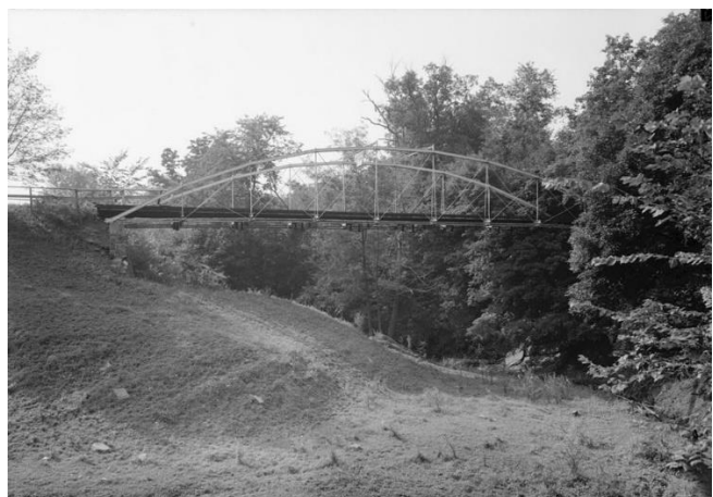
Figure 26: A Whipple bowstring truss bridge in the US, image undated. Source: Structure Magazine, https://www.structuremag.org/?p=7899
