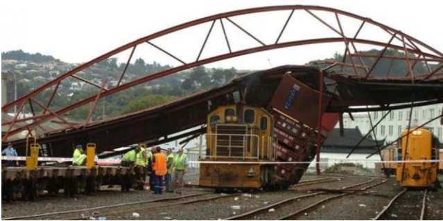
Figure 29: The Dunedin Rail Station footbridge after being hit by a train in 2008. Source: Otago Daily Times
