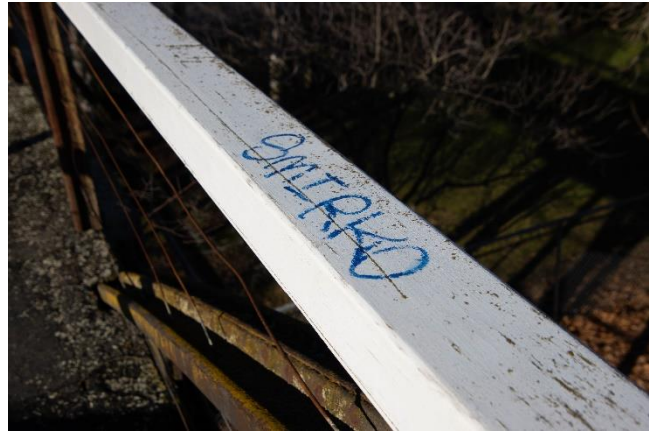
Figure 101: Graffiti damage to the timber handrail.
