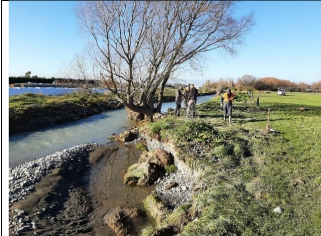
Above: June 2021, Looking downstream from right bank: flood damage to Mt Harding Creek at H Rooney's farm. The true left bank was scheduled for riparian planting (visible here, with white-wrapped baleage line beyond).
