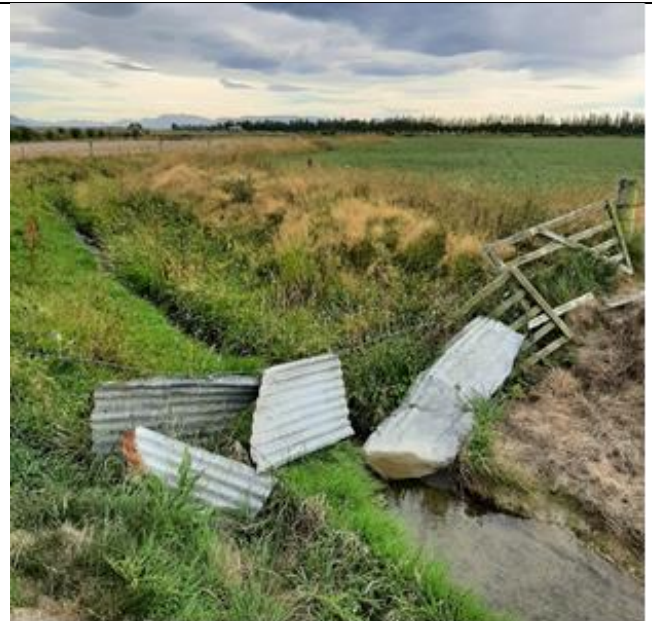
Ad-hoc fencing example at a farm boundary Creek crossing.
