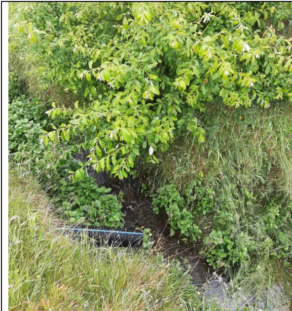
Picture above left: Novaflo -type plastic drain pipe installed to drain dairy paddock sub-soil direct to Washpen Creek (in upper Mt Harding catchment, where our water testing showed high levels of nitrates and detectable phosphates).
