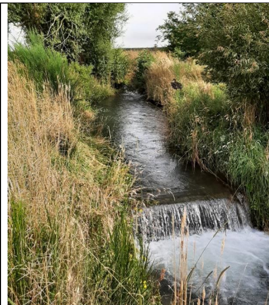
Example above of small in-stream step weir (photo 2 Feb 2021). There are many weir steps of around this size: see list in Appendix 2.
