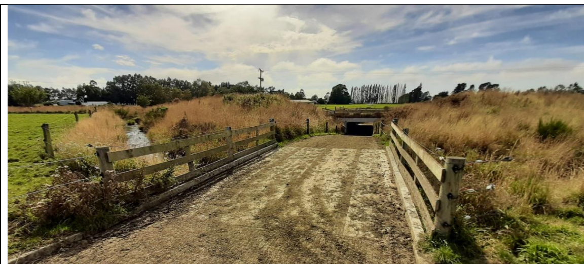
An example of 'good practice' stream stock-bridging on a dairy farm, where fencing prevents stock access to Mt Harding Creek and the bridge approaches are either level or sloping away from the water, and its concrete track edges are raised (bunded) to help manage animal manure and urine.
