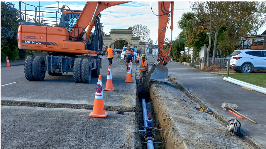
Crew from contractors ACL have been replacing water mains in McDonald Street, Methven.
