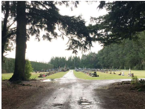
A. GRAVEL DRIVEWAY WITH PONDING AND POT HOLES
