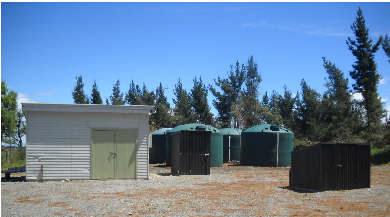
Figure 14 - Hinds Water Treatment Plant
