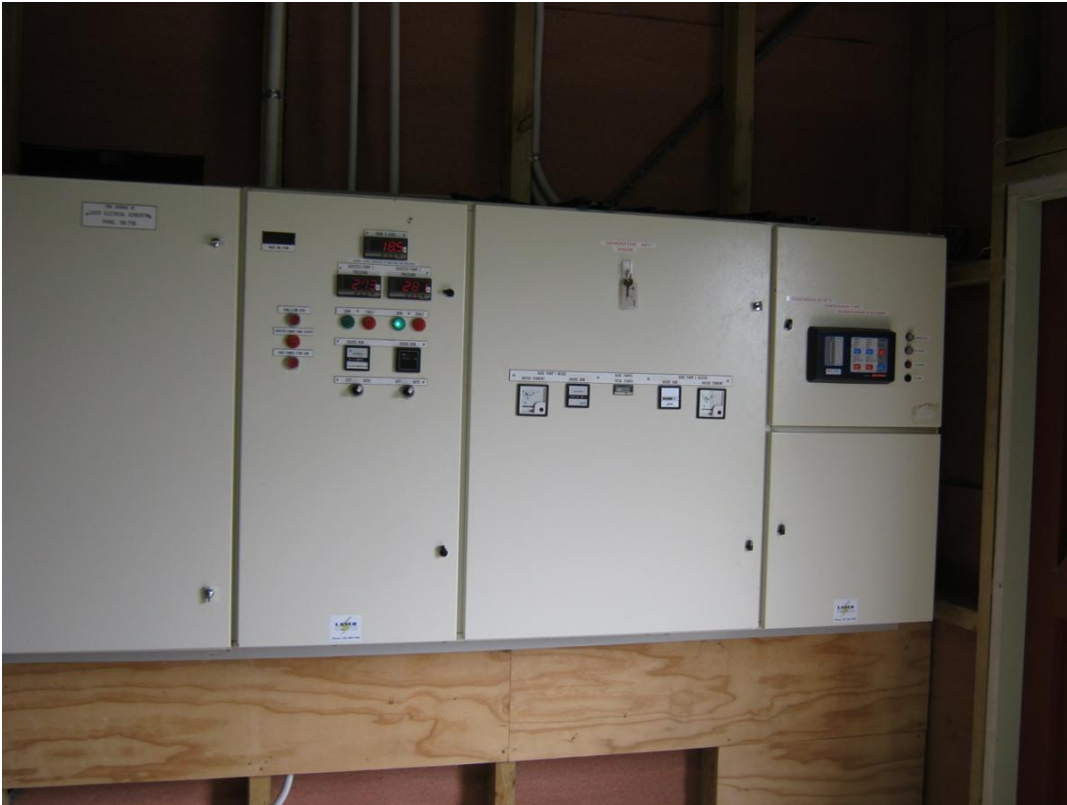
Figure 13 - Electrical and Control Equipment
