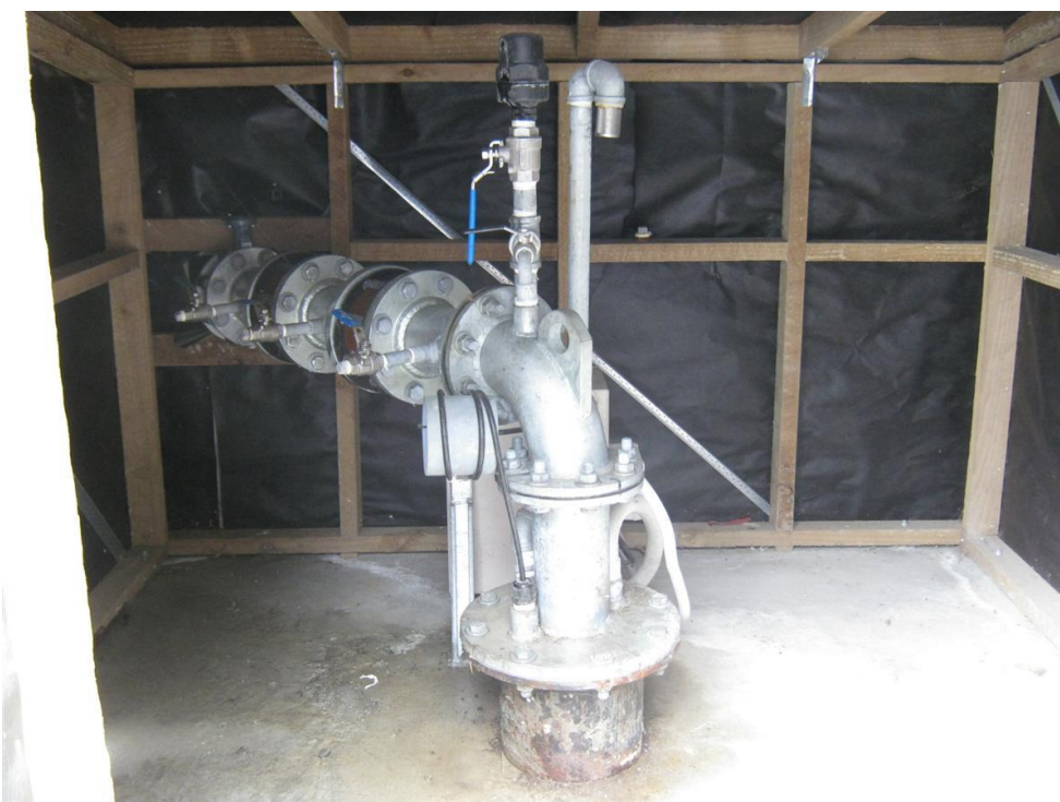
Figure 6 – Wellhead (Inside)
