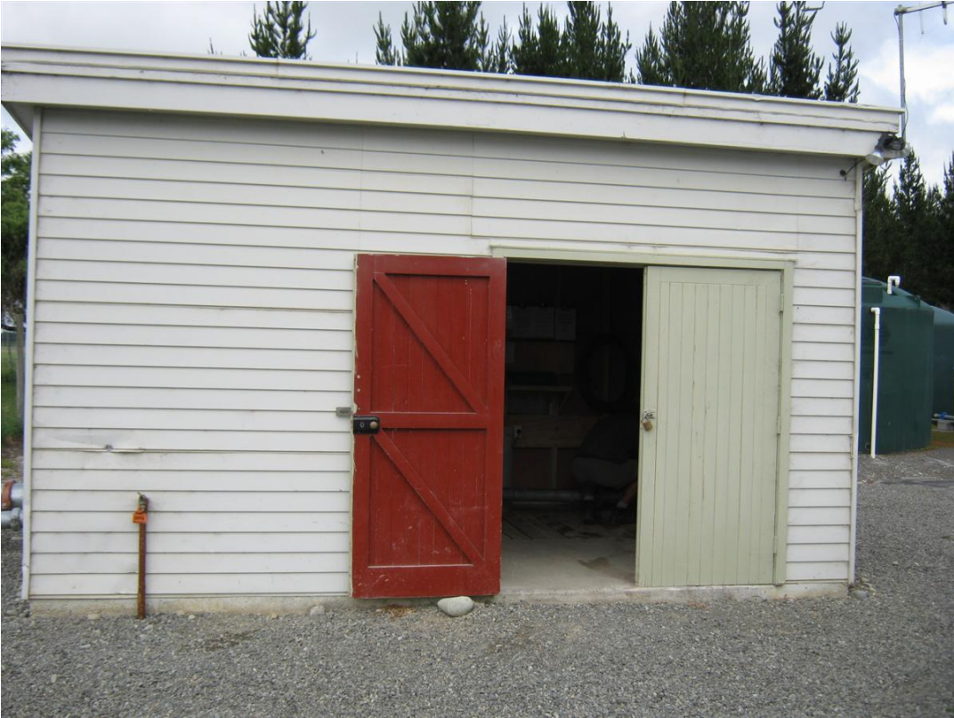
Figure 9 – Pump Station and Treatment Building
