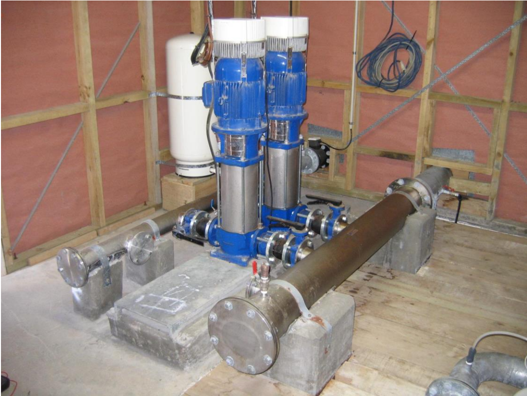
Figure 8 - Water Distribution Pumps
