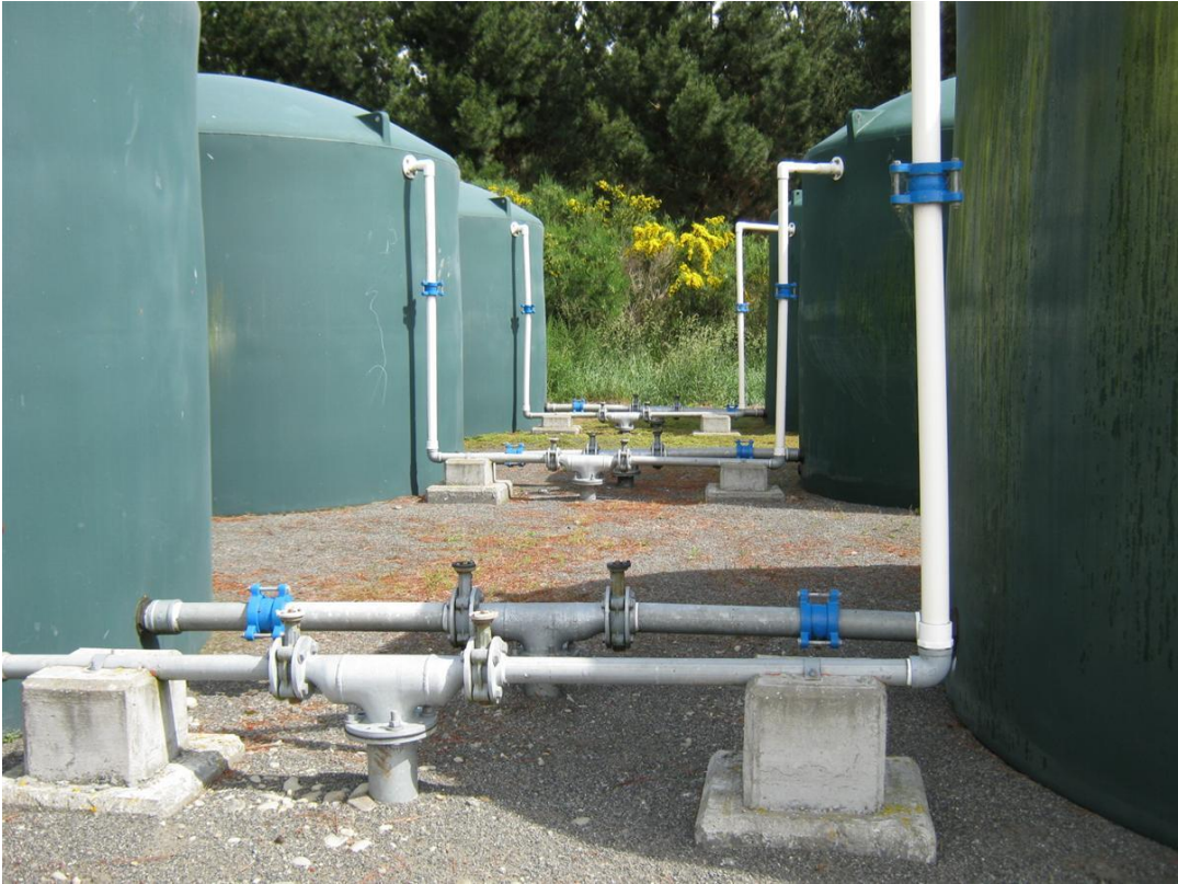
Figure 7 - Six 30m 3 PE Supply Reservoirs
