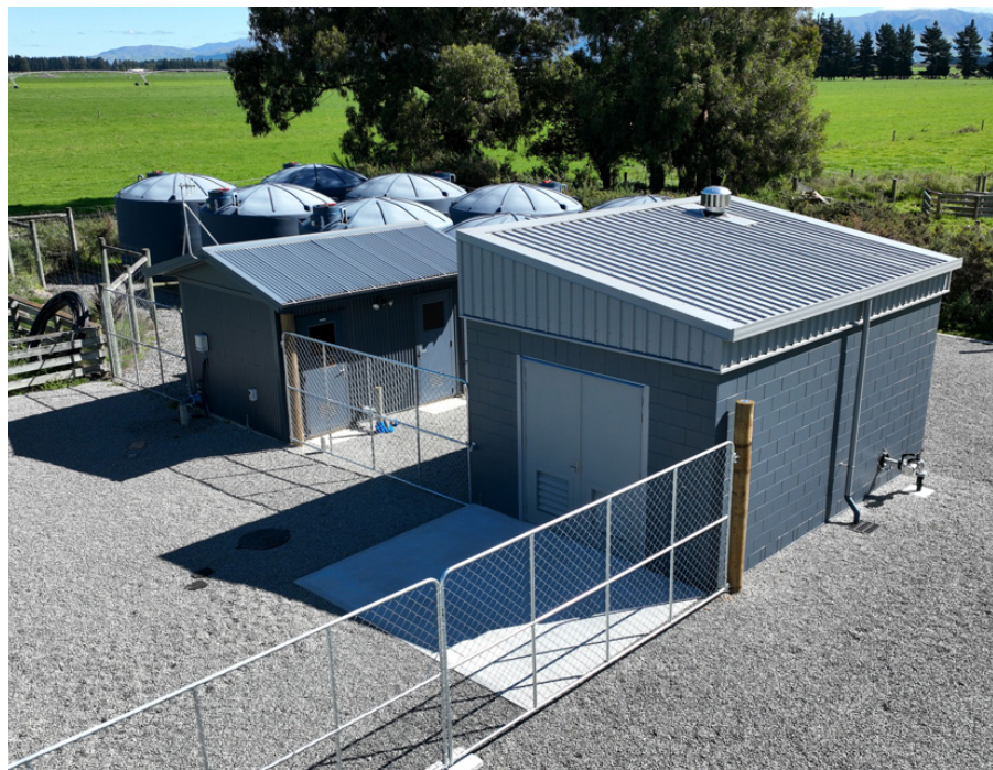
Mayfield's water treatment plant has a new building to house new filtration and UV disinfection equipment.
