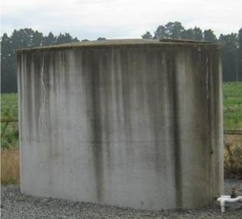
Figure 8 - 23 m 3 Concrete Tank
