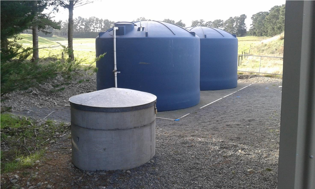
Figure 7 - Two 30m 3 PE tanks and Wellhead Chamber
