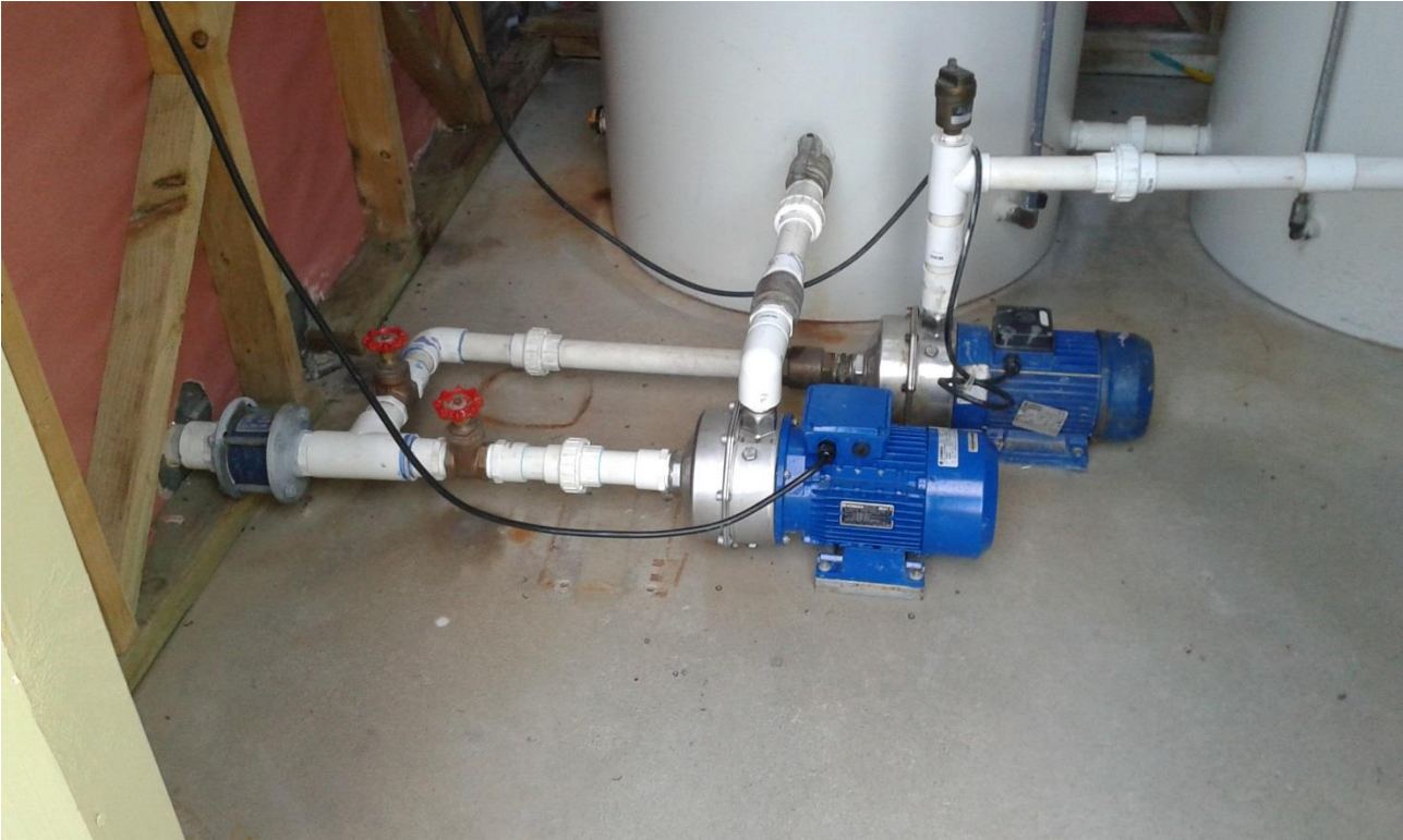
Figure 9 - Lowara Booster Pumps
