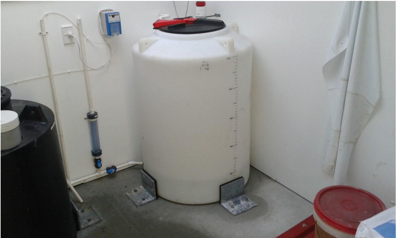
Figure 11 - Chlorine Tank
