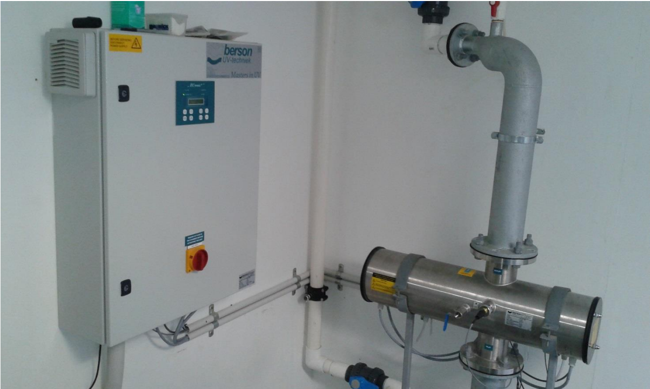
Figure 10 - UV Treatment & Telemetry
