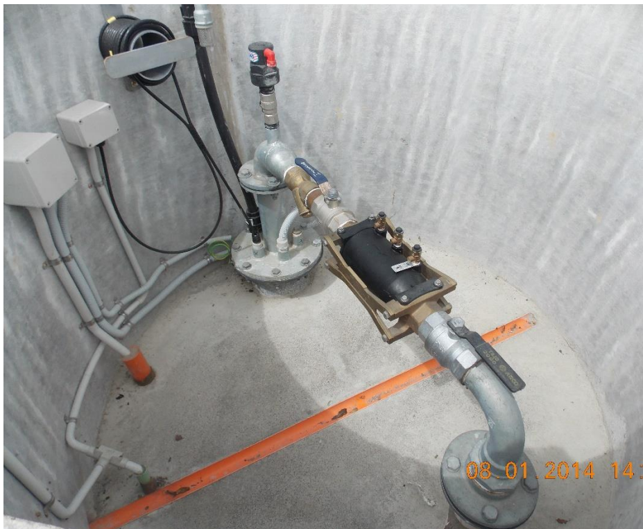
Inside of Borehead Chamber
