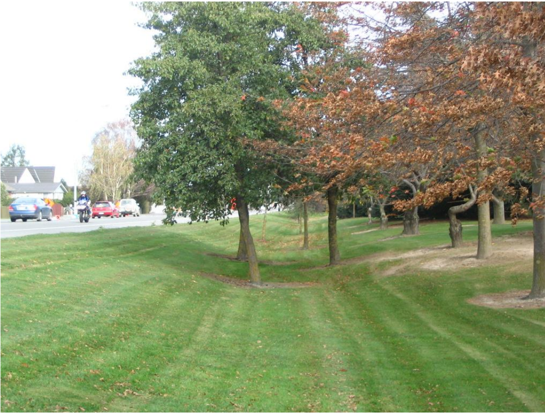
Figure 3 – Example of a road side swale adjacent to State Highway 1 in Tinwald
