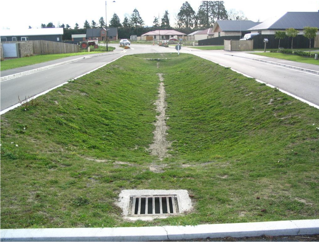
Figure 2 – An example of an infiltration basin / swale located within a central median
