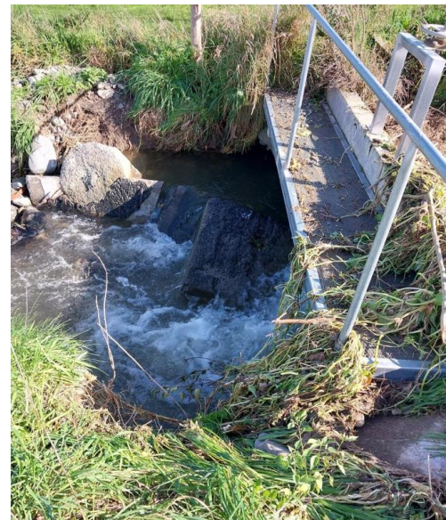
Damage to stormwater gate post event
