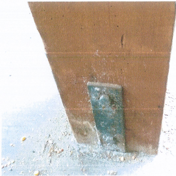
Photo 5: Post connection at base
