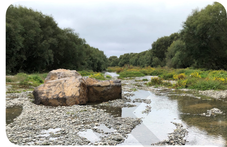
Rocks installed in the lower Hekeao / Hinds river create a better environment for freshwater fish.
