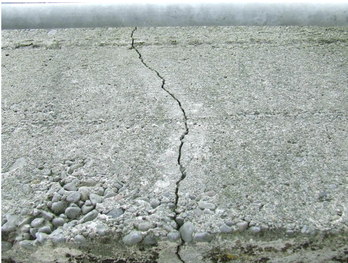
Photo 15. Chimney – Vertical crack on southwest side.
