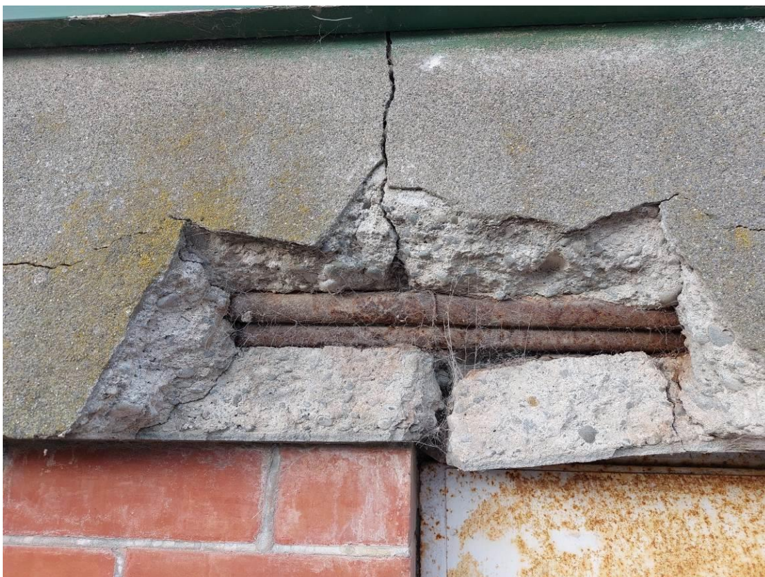
Photo 19. Building 1. – Spalled concrete on bond beam on grid H.
