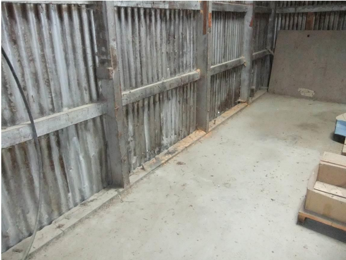
Photo 44. Building 3. - Dust from borer.
