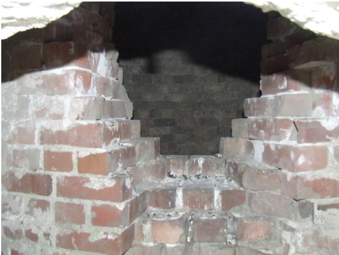
Photo 17. Chimney – Hole in southwest side. View of internal brick flue.
