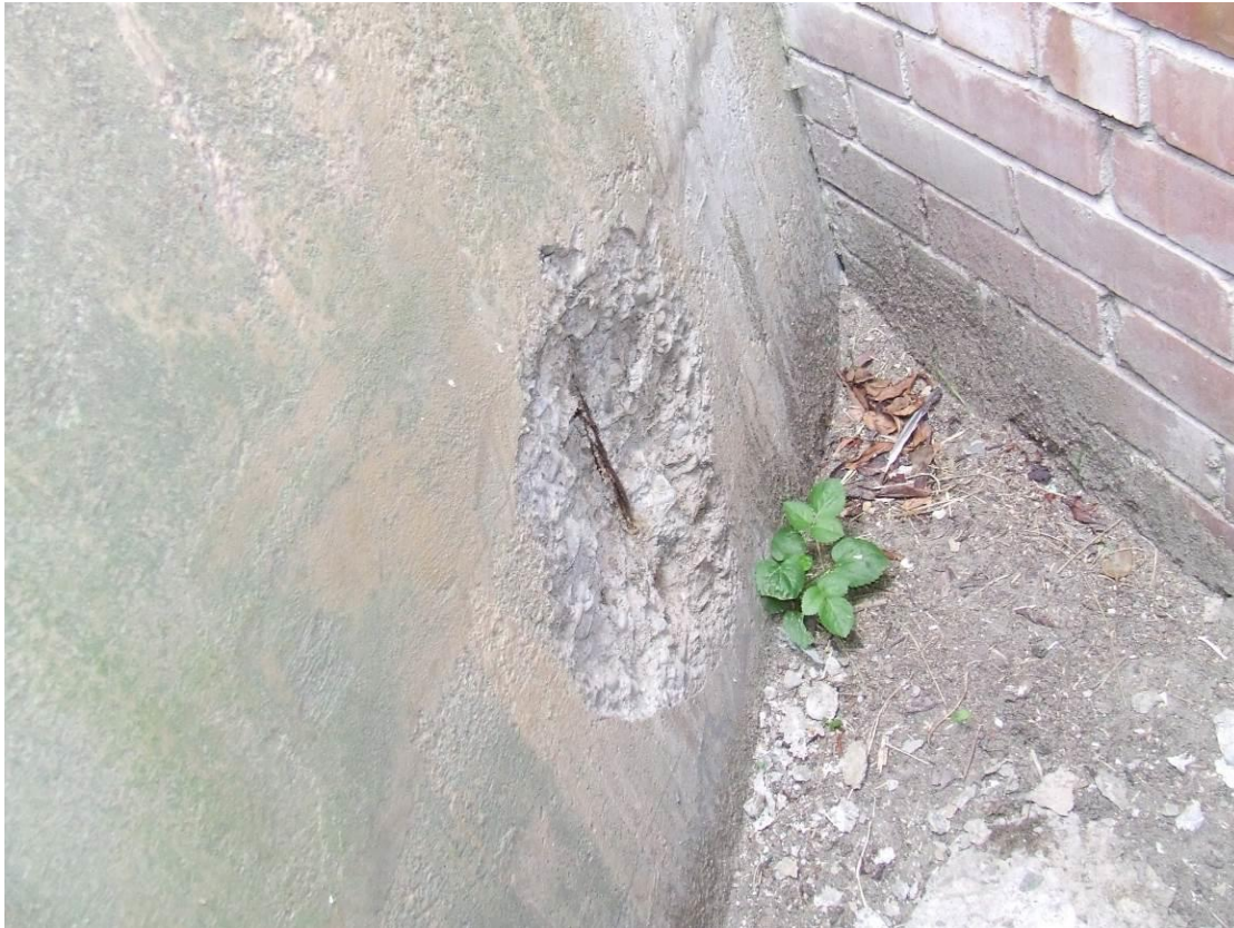
Photo 16. Chimney – Spalling on northeast side.
