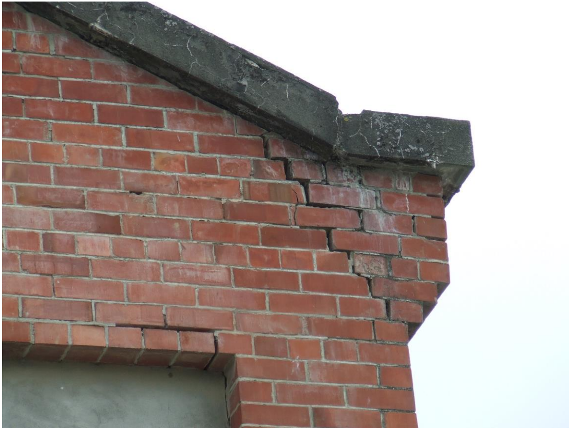
Photo 10. Eaves brickwork and coping damage on Building 1 gable end west corner.
