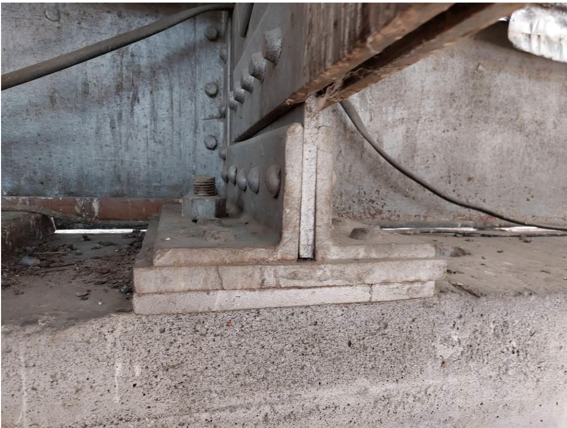
Photo 27. Building 1. – Main Hall truss eaves support.
