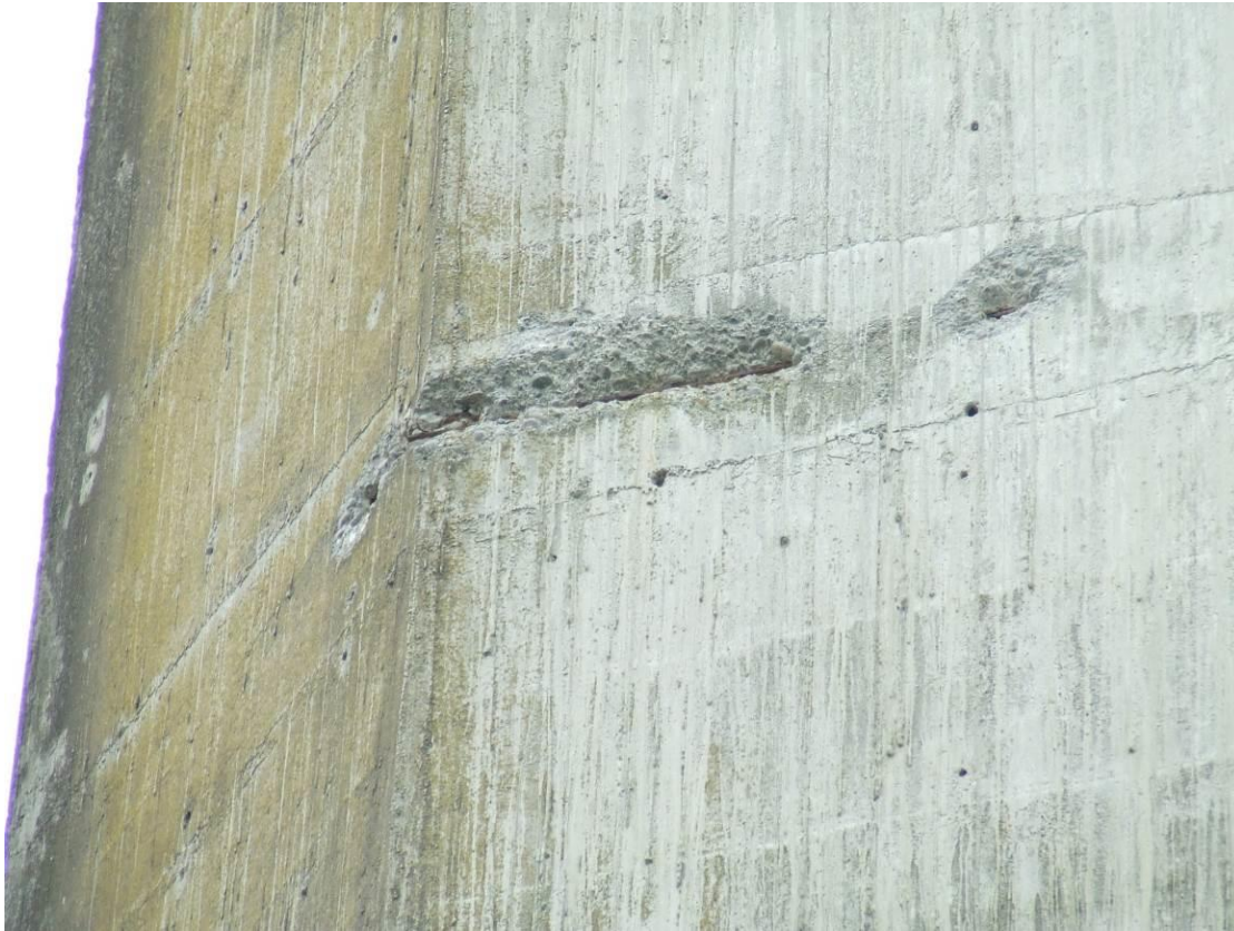
Photo 12. Chimney – Spalling due to reinforcement corrosion.
