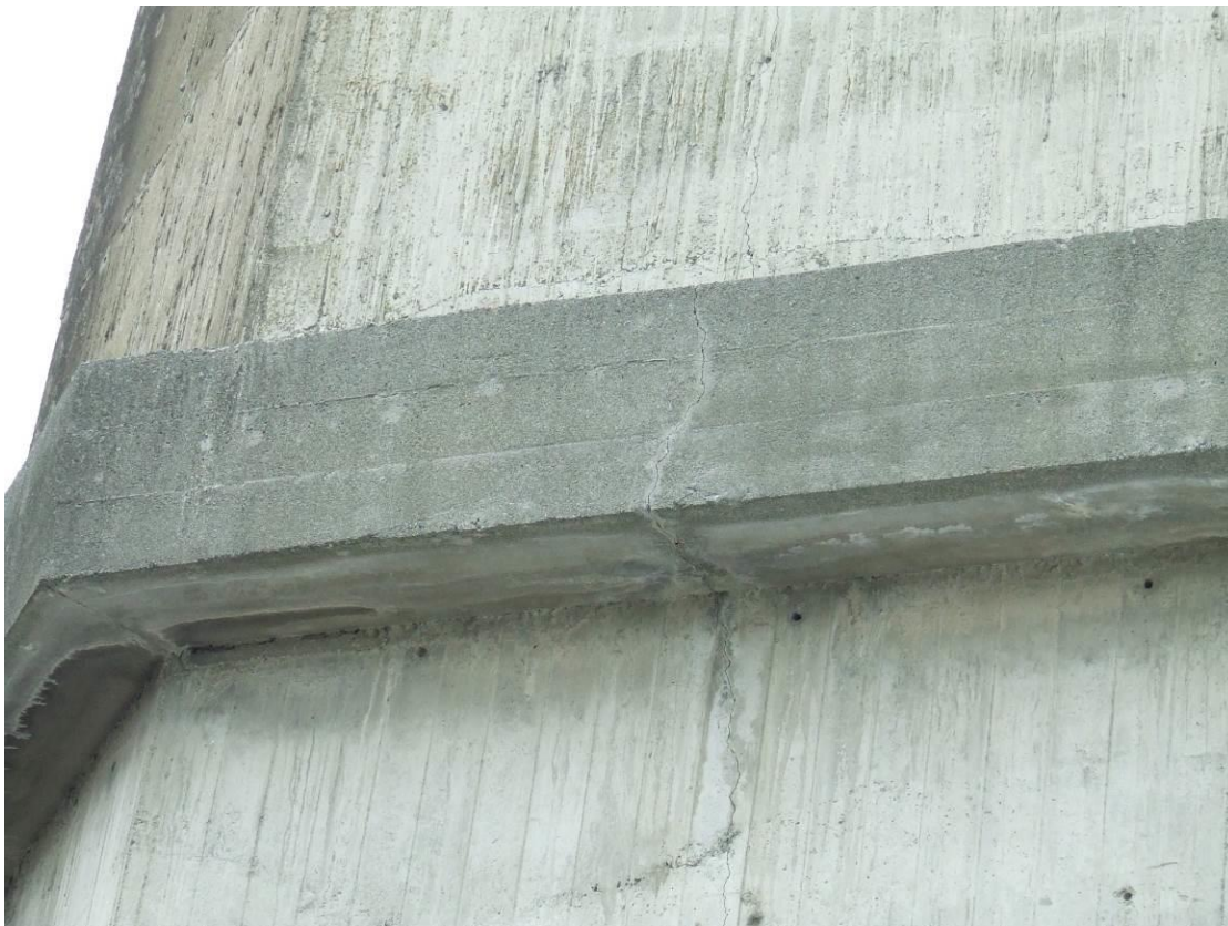
Photo 13. Chimney – Vertical crack on northeast side.
