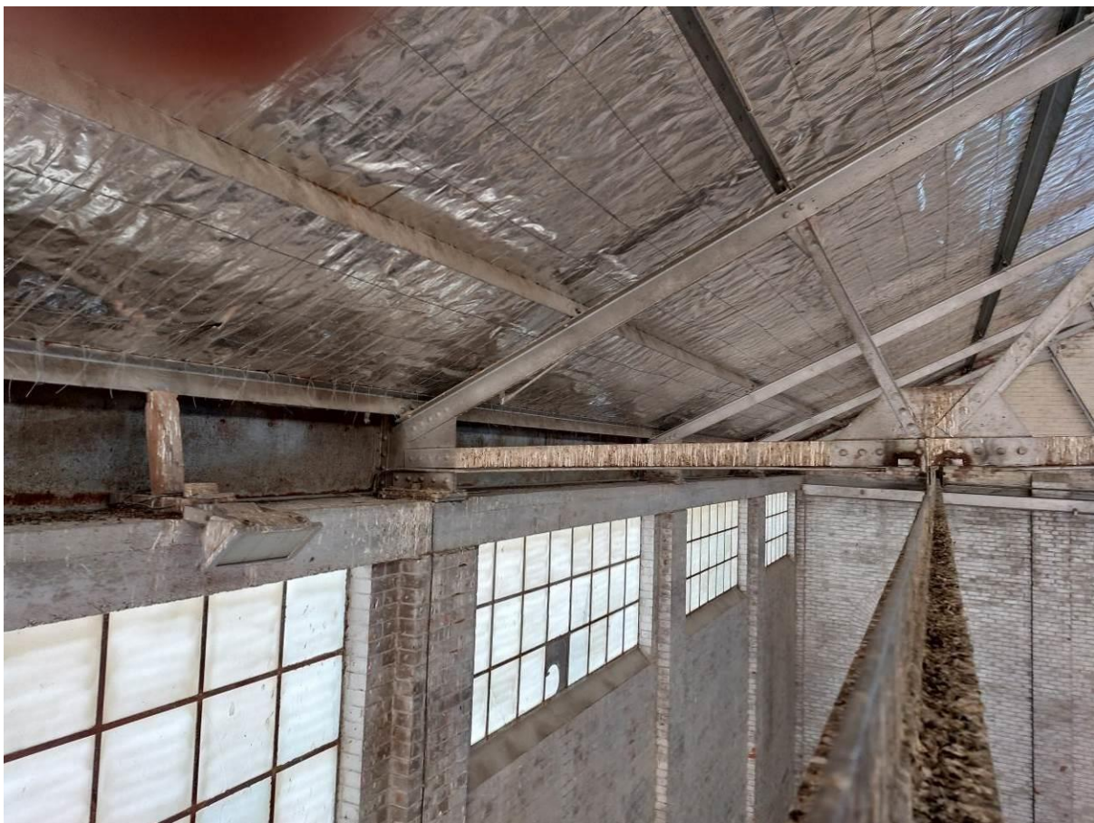
Photo 25. Building 1. - Main Hall truss connection to bond beam.
