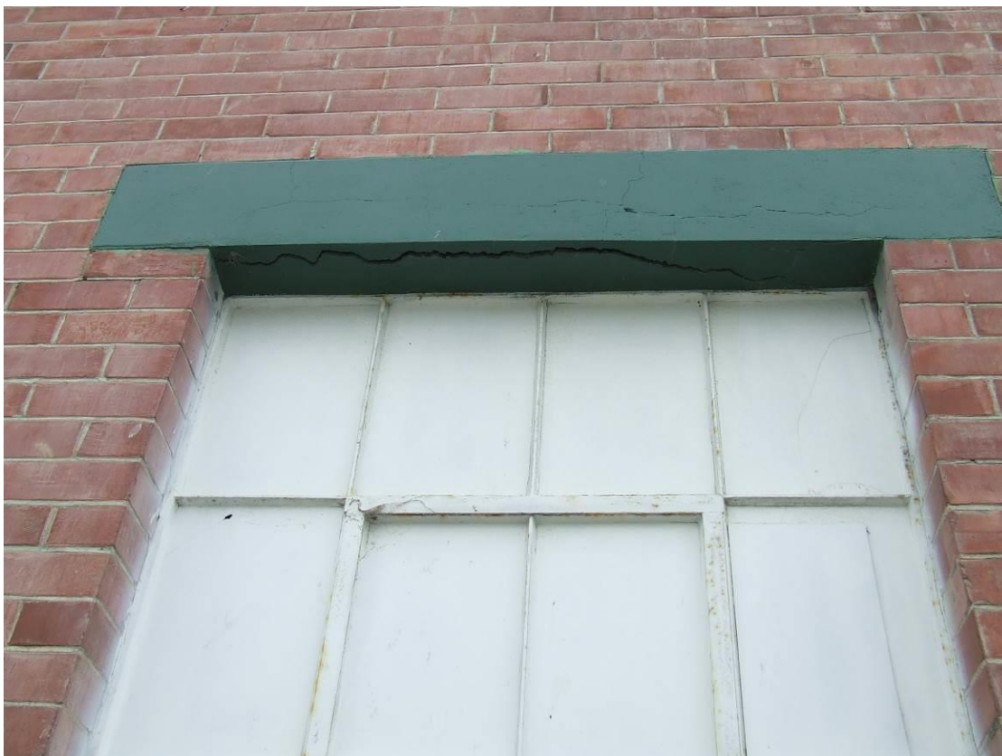
Photo 11. Lintel cracking due to reinforcement corrosion on Building 1 Northeast Elevation.
