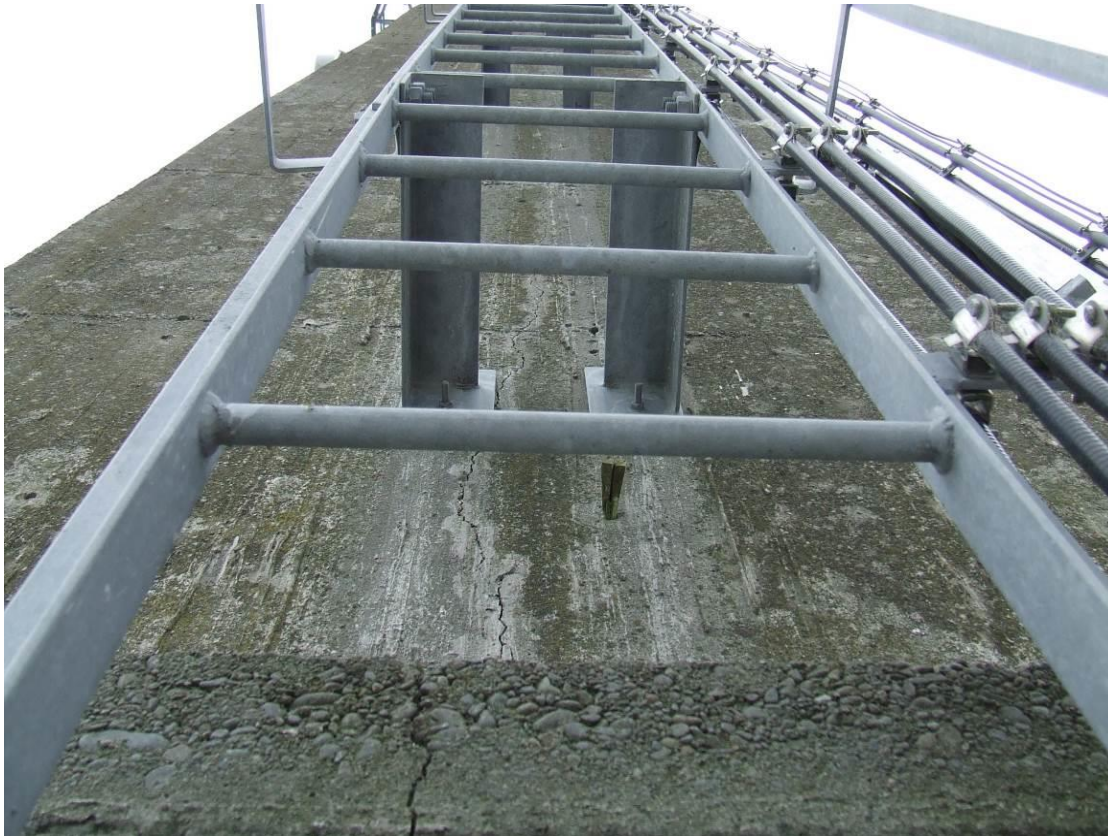
Photo 14 Chimney – Vertical crack on southwest side.
