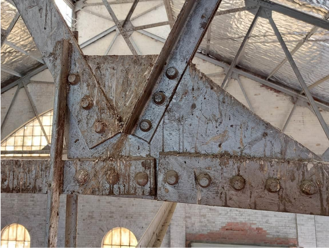
Photo 26. Building 1. – Main Hall typical truss joint.
