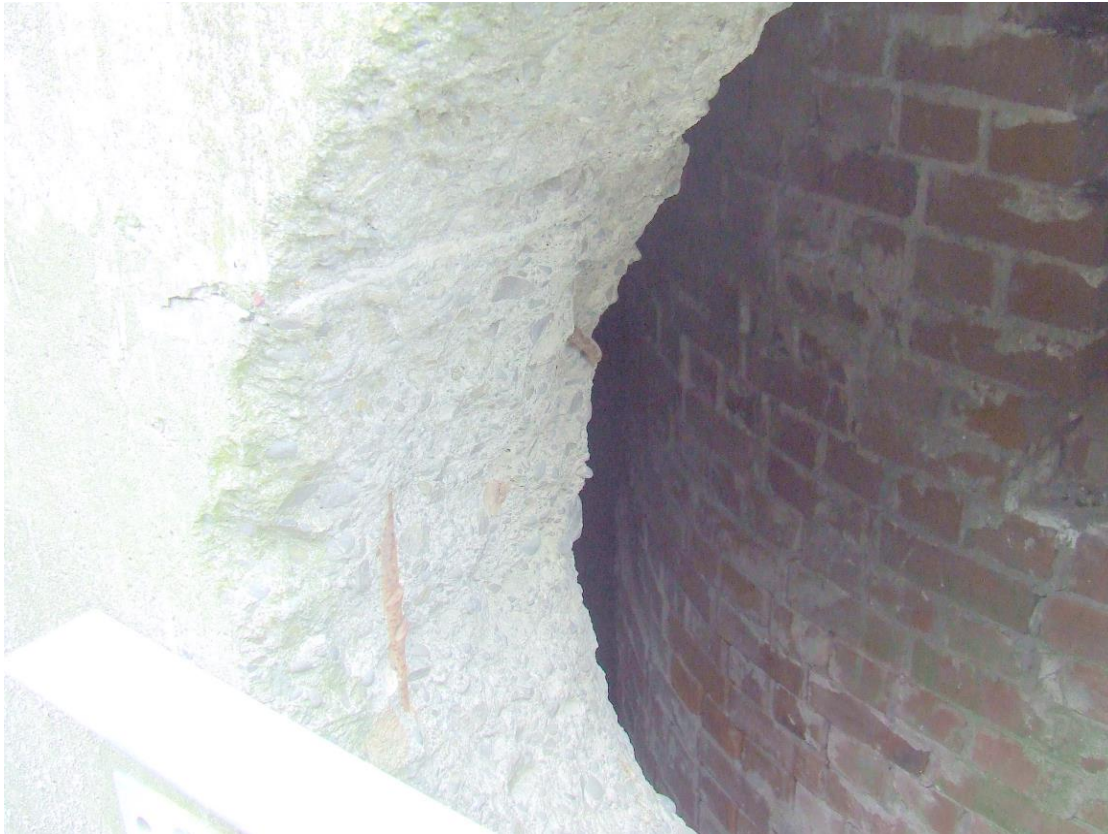
Photo 18. Chimney – Hole in southwest wall.
