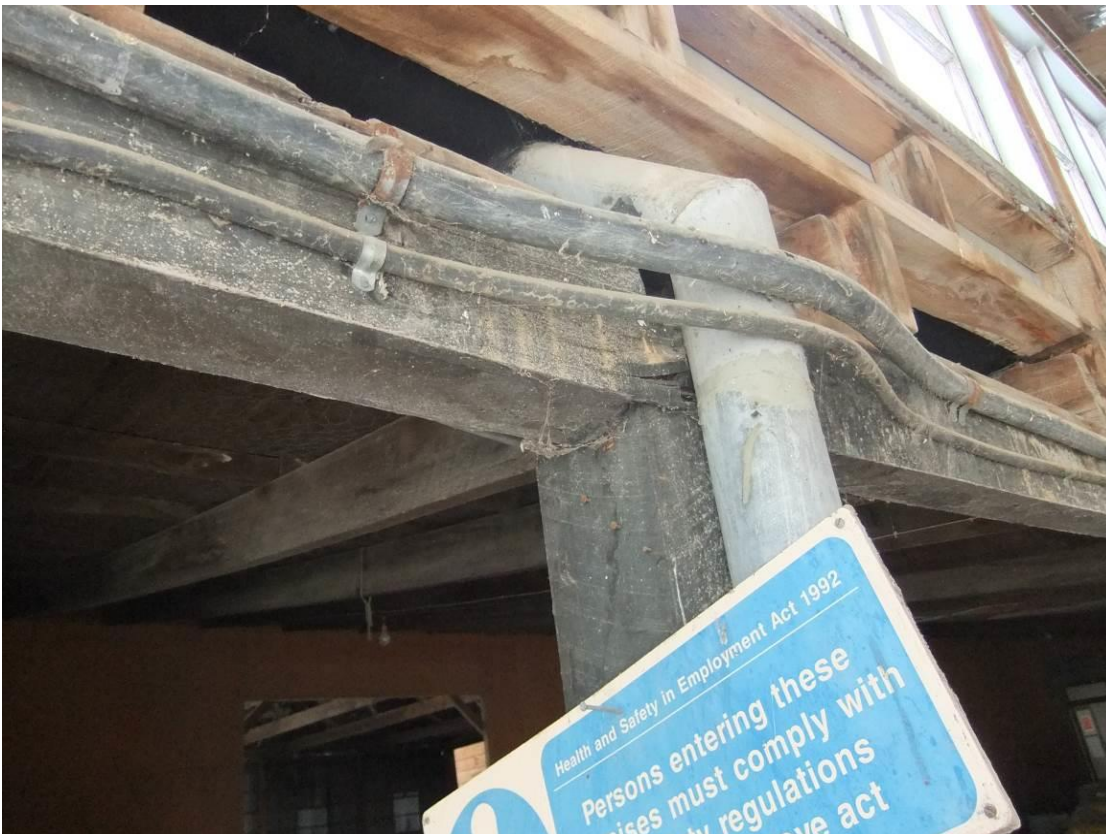
Photo 47. Building 2. Timber beam rotten over post due to downpipe leak.
