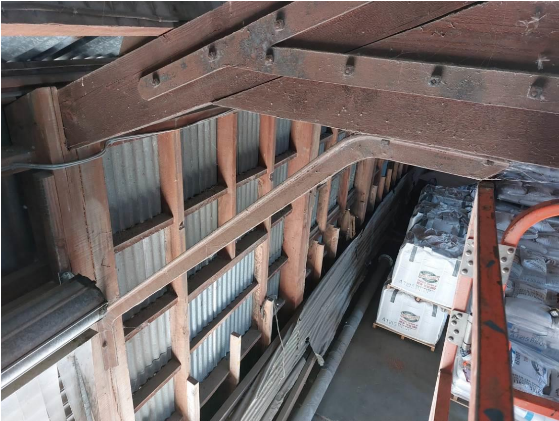
Photo 40. Building 2. Truss connection.
