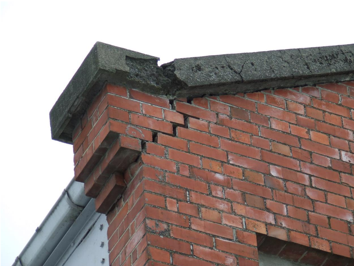
Photo 9. Damage to gable end brickwork and coping on Building 1 west corner.
