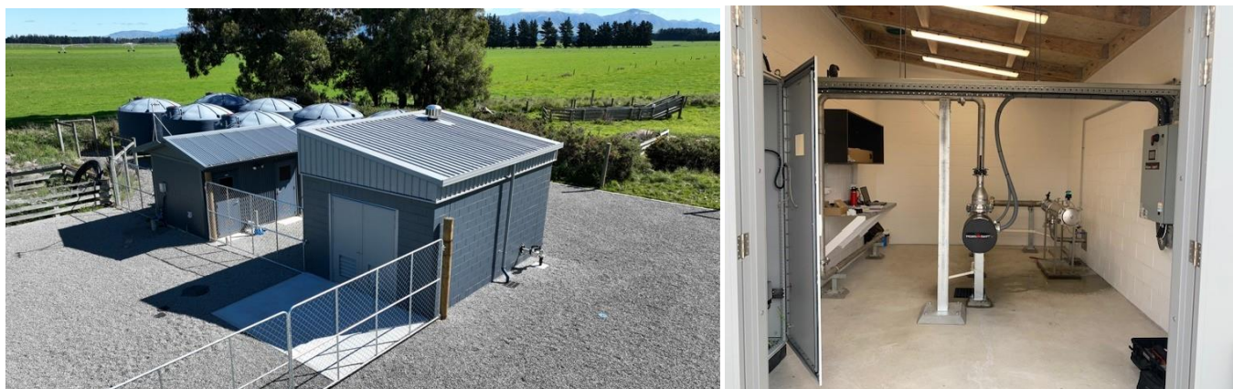
Figure 1. Mayfield drinking water plant (left), and UV equipment (right).
